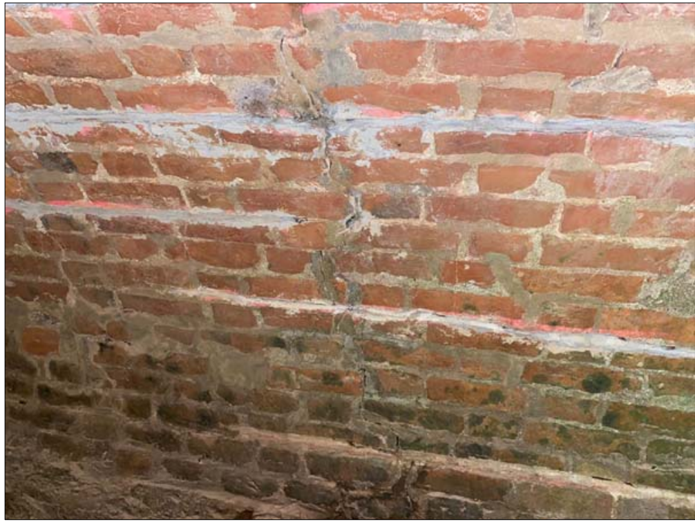
Photograph-1-Cracking within barrel with evidence of longitudinal stitching
