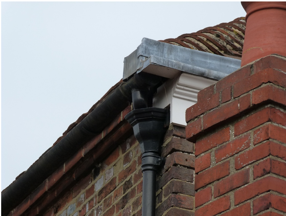
end of lead lined timber gutter where overflow to be fitted.
