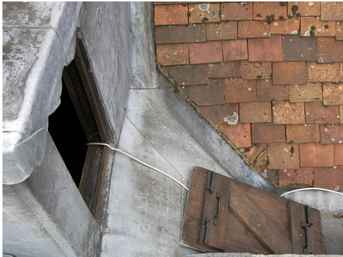
cupola base and cladding to pediment and into gutters either side
