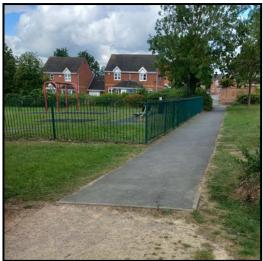
The existing safety surfaces within the fenced off play area is wet pour that requires replacement with rubber mulch surface in suitable locations of the play equipment.
