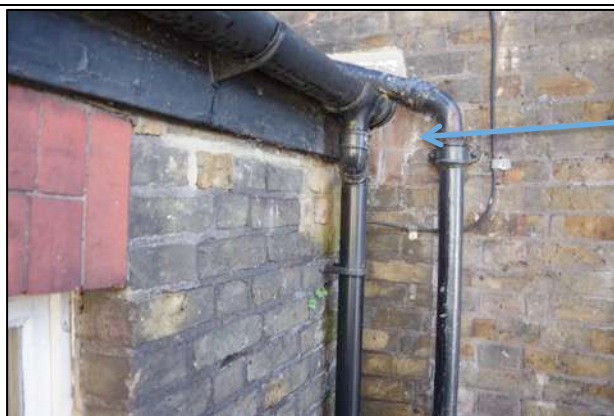
Remains of an arch where the toilet extension has been built onto the rear wing
