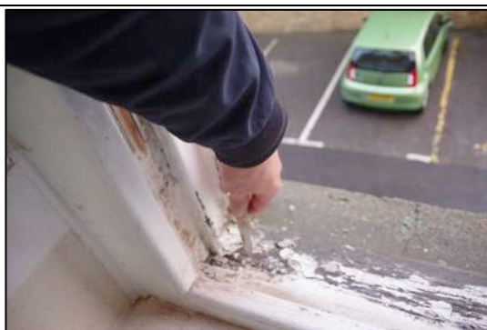
Example of a timber sill being checked with a knife for firmness
