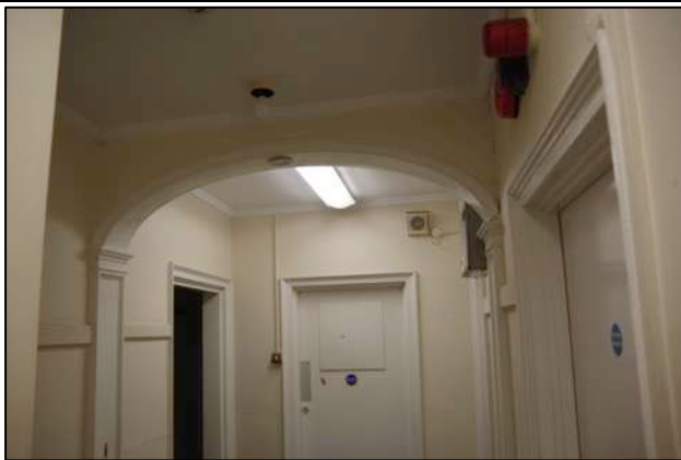
Elliptical arch between the spine walls
