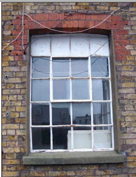
The 'Hopper' window at the rear Watch Room
