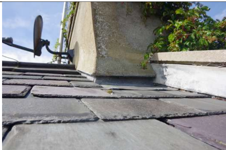
Example of weathering detail at bottom of a stack
