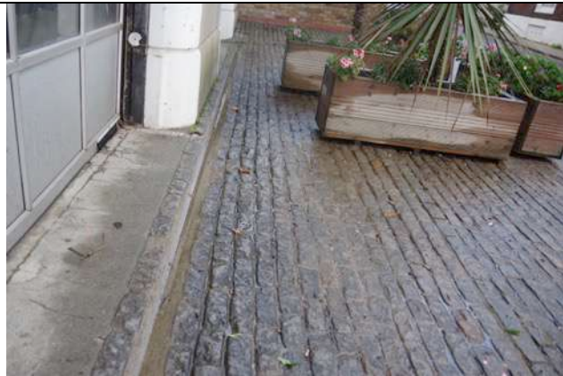
Gully formed at the front to the roller shutter doors
