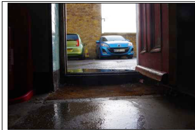
Rainwater ponding at the side entry door
