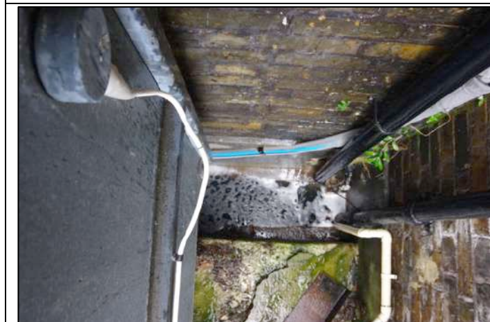
The downpipe that services the rainwater from the flat roofs and domestic wastes discharging over a blocked drain
