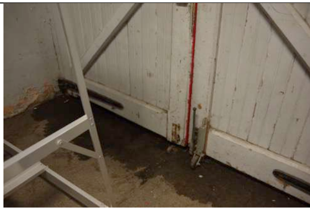
Rainwater penetrating into the carriage entry
