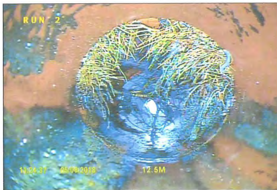
Photo: 3_3_14_A.jpg 12.5m, Roots, mass at joint, 40% cross-sectional area loss
