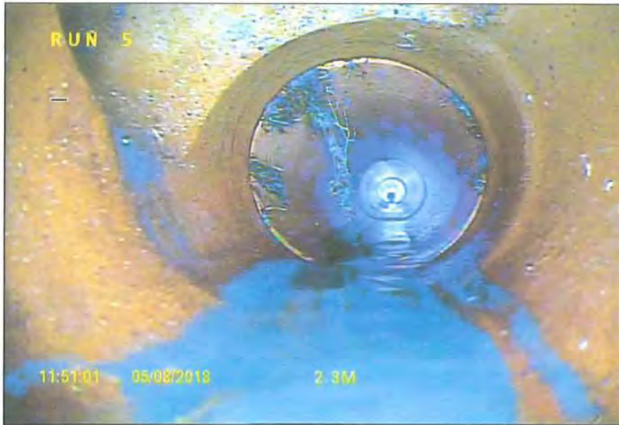
Photo: 6_6_33_A.jpg 2.3m, Roots, mass at joint, 5% cross-sectional area loss
