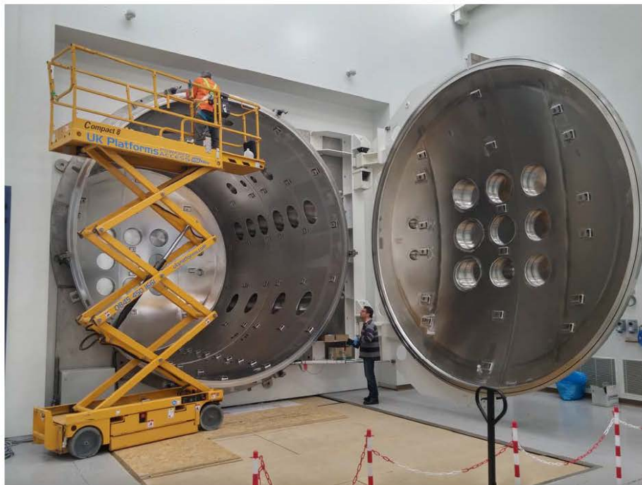
Figure 1: STC-2 vacuum chamber during installation
