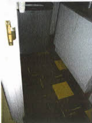
Asbestos floor tiles within basement kitchenette B16
