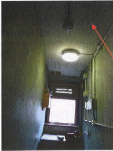
AIB ceiling panel in boiler room B15
