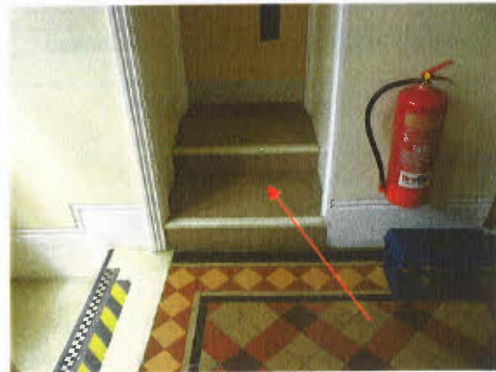
Asbestos floor tiles on steps leading to annexe Rm 9
