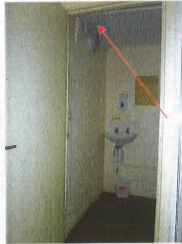
AIB ceiling panels within shower room and WC
