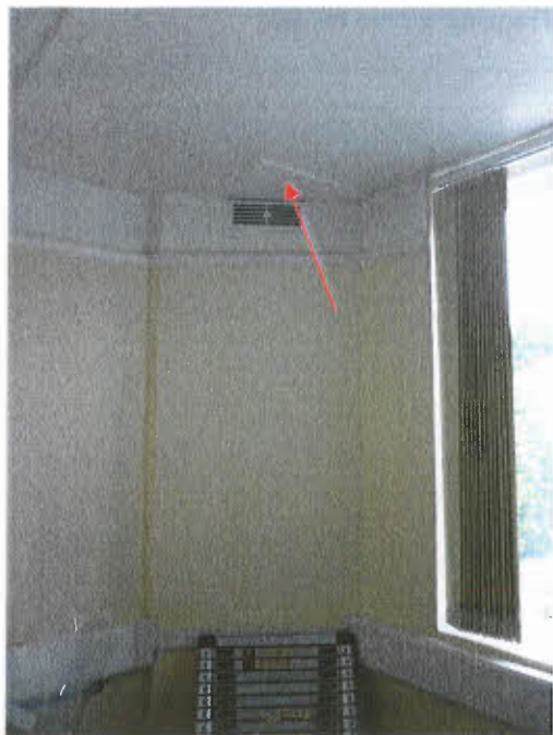
Asbestos cement panel to wall in post box of annexe reception
