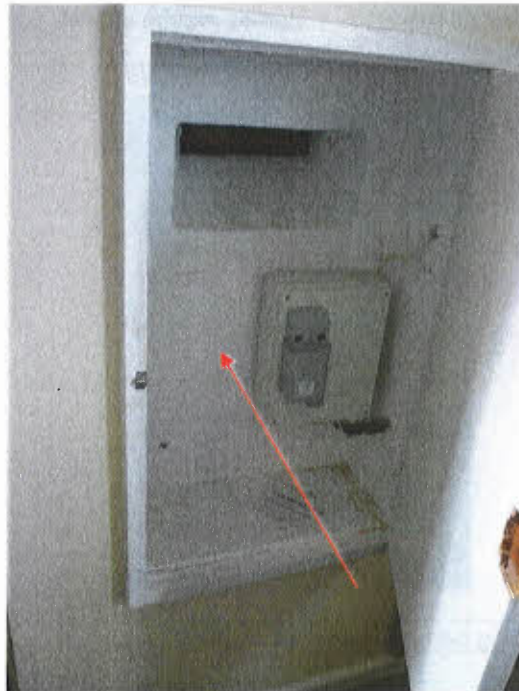
Asbestos Cement panel to ceiling in annexe interview room
