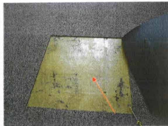
Non asbestos floor lino found beneath floor coverings in some rooms.
