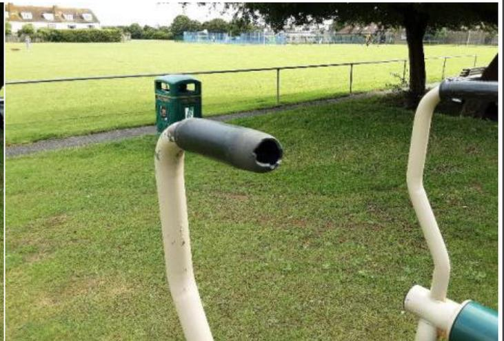
**Finding:** One or more handgrip(s) are damaged or missing.
