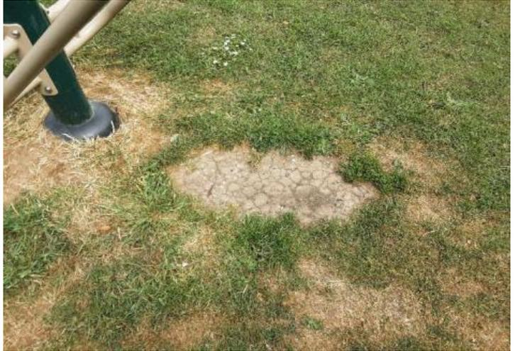
**Finding:** The grass mats are silted up, the soil is compacted and the area will become very slippery when the soil is wet.
