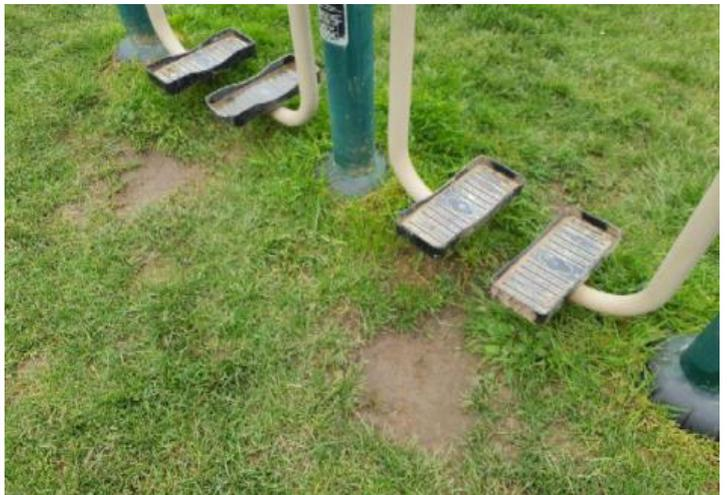
**Finding:** The grass mats are silted up, the soil is compacted and the area will become very slippery when the soil is wet. **Action:** Reinstate as required
