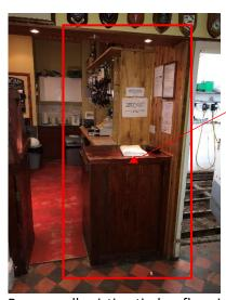
Area to be removed and reinstated. Note the floor need to be remove and joists spliced as they run through to beer room and kitchenette and bear on sleeper wall.
