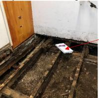
Existing sleeper wall to be rebuilt. New wall to retain new concrete floor and support bar area floor joists on new joist hangers.
