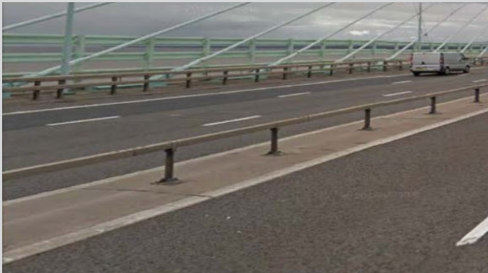
Figure 2: Existing steel central reservation barrier
