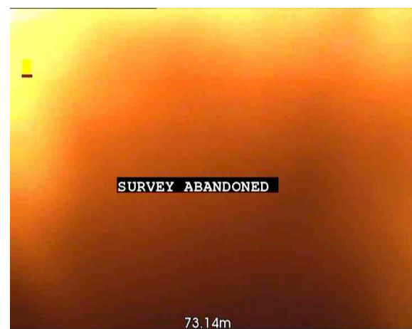
4, 00:04:42, 73.14 m Survey abandoned, Unable to continue
