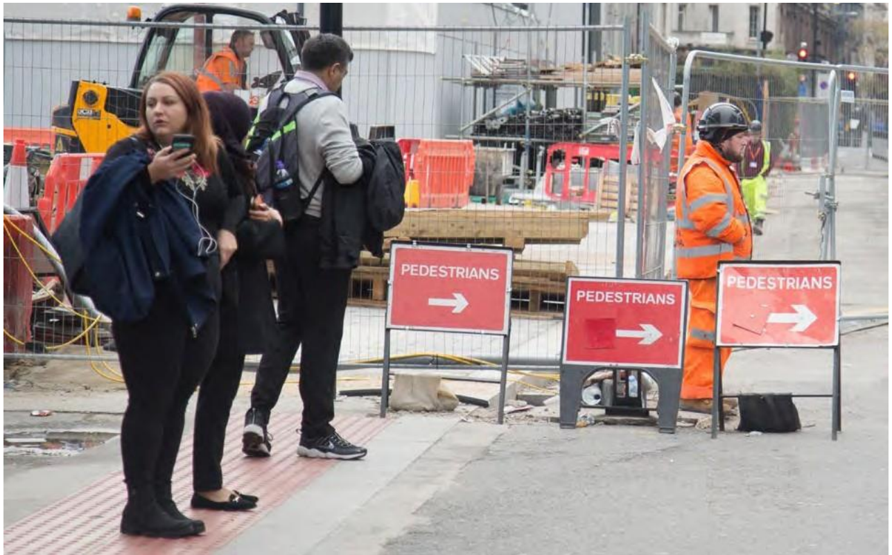
Marshals can help maintain a safe system of work and assist pedestrians
