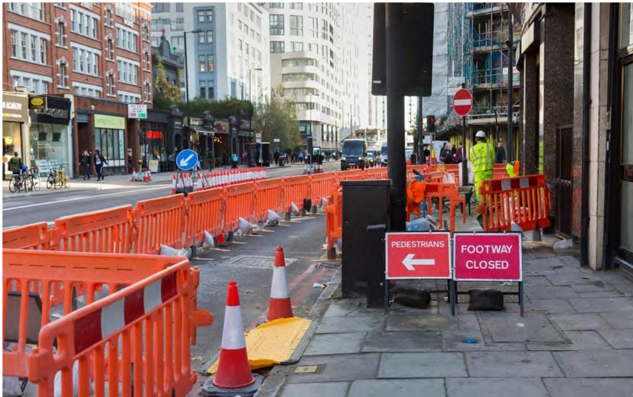
Closed footway with temporary walkway in carriageway
