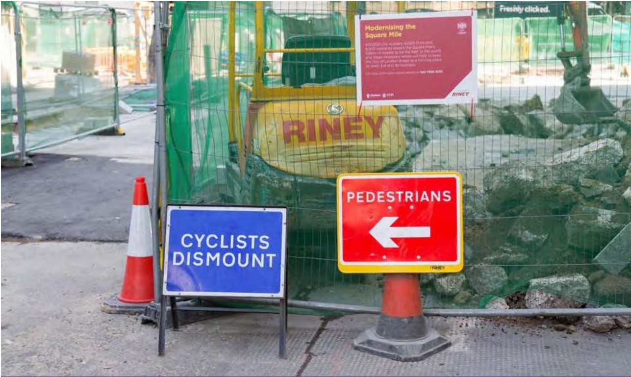
Bad practice: designers must ensure they use the right signs and choose the right colours to ensure traffic management is compliant and consistent
