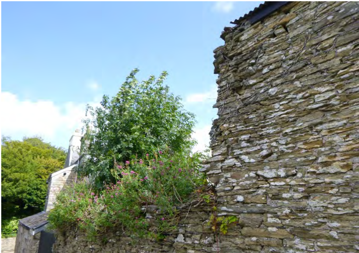
Photograph 49: Unstable boundary wall along Varley Lane approximate NGR 224943, 064470.
