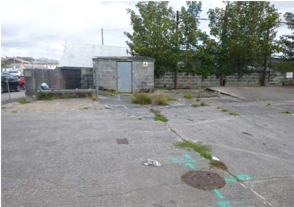
Photograph 25: Vehicle and stock container washing facility, note raised concrete platform, underground services and oxidised metal wash posts.
