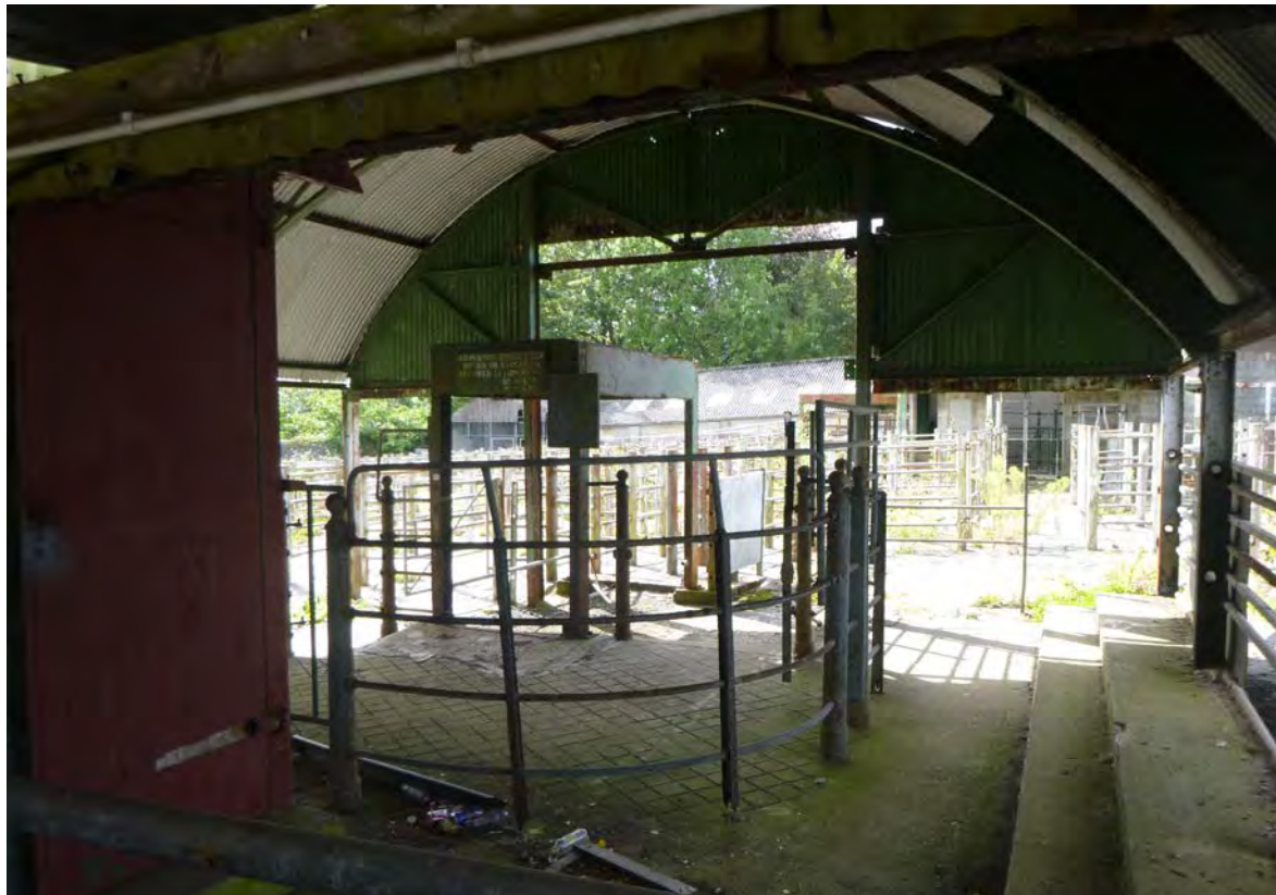
Photograph 33: Outbuilding, cattle yard. Note corroded steel supporting beam and suspected asbestos roof.
