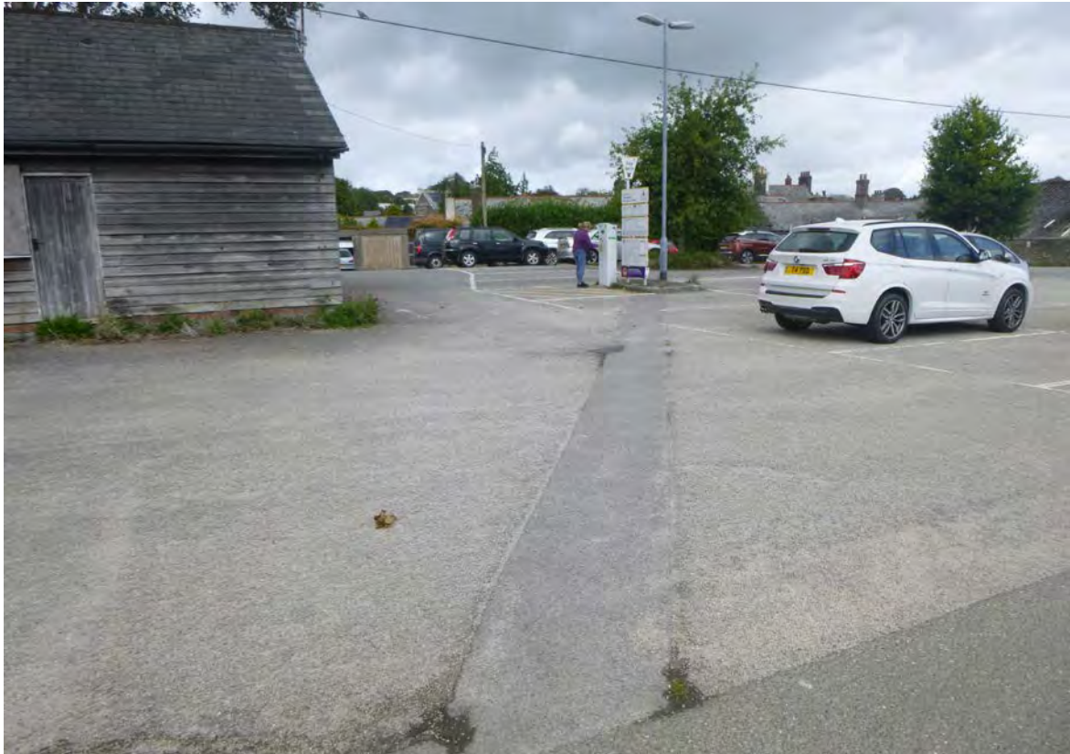
Photograph 45: Reinstatement scar illustrating abundance of buried services.
