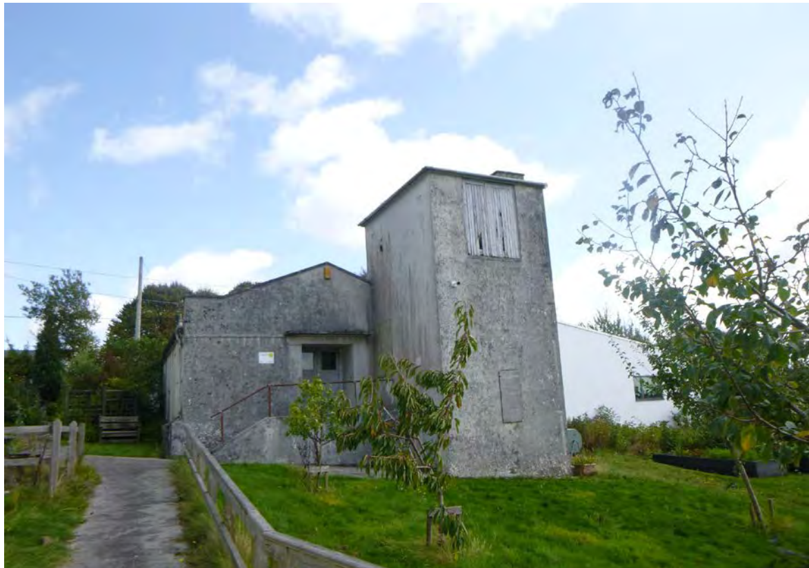
Photograph 9: Water tower (NGR 224894, 064366), suspected asbestos roof and anecdotal evidence of gas powered boiler inside.
