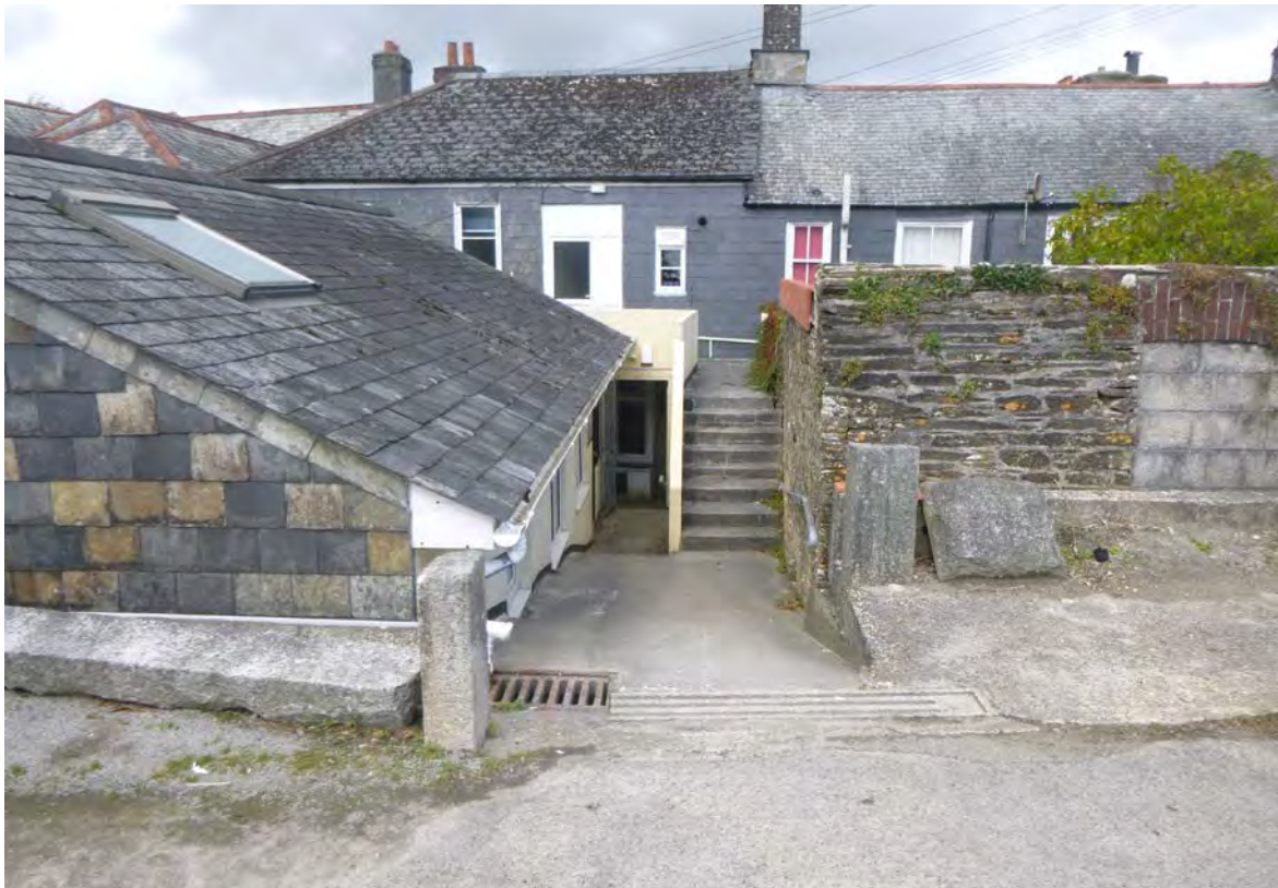
Photograph 43: North-west car park boundary, note small drain and sloping concrete ramp giving rise to potential localised flooding events.
