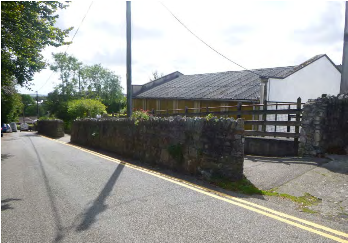
Photograph 13: Historical granite wall, note outbuilding with suspected asbestos roofing (NGR 224912, 064368).
