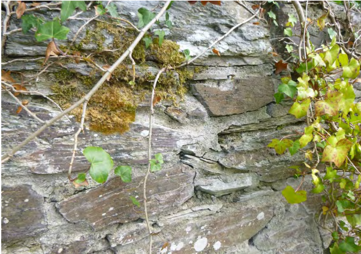
Photograph 21: Cracking of rendering observed in western boundary retaining wall.
