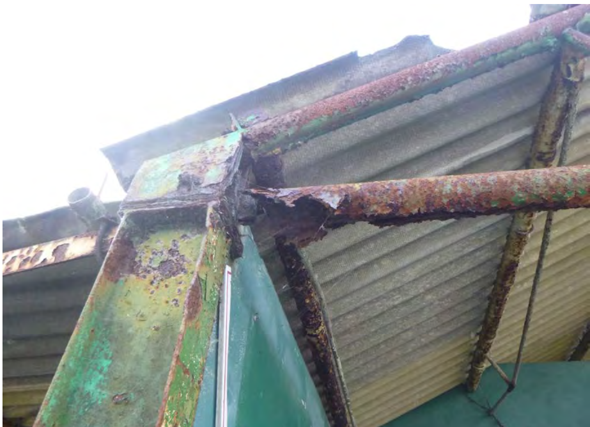
Photograph 34: Cattle yard. Note corroded steel frame. NGR 225040, 064368.
