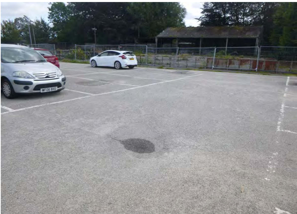
Photograph 22: Localised shallow depressions, western car park surface.
