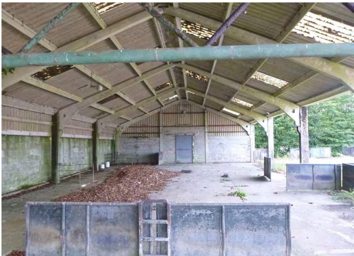
Photograph 24: Sheep yard (NGR 224943, 064359), note concrete floor and steel frame.
