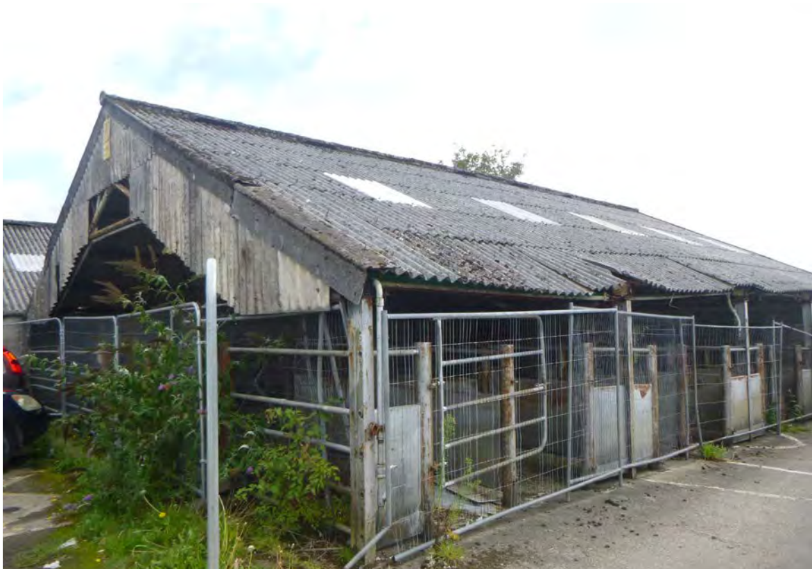
Photograph 29: Cattle yard barn, note suspected asbestos roof (NGR 225055, 064377).
