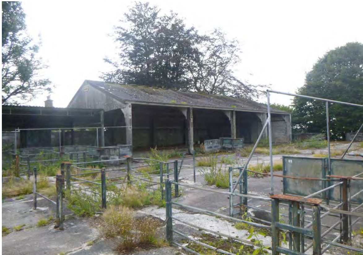
Photograph 23: Sheep yard (NGR 224943, 064359), suspected asbestos roof.
