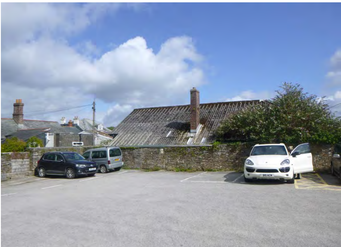
Photograph 42: Suspected asbestos roof at NGR 225003, 064430.
