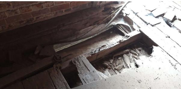
2.2.3 Clear debris from the decayed southeast <u>staircase</u>, above and below, and install temporary propping from ground floor and temporary tread boards, to facilitate occasional accompanied access.
