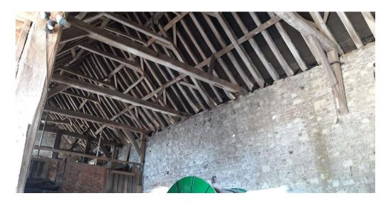
2.1.9 At the Barn's West end internally, prop the two western N-S principal floors beams supporting the gallery platform at the north bearing ends, with Accrows based on the solid floor.
