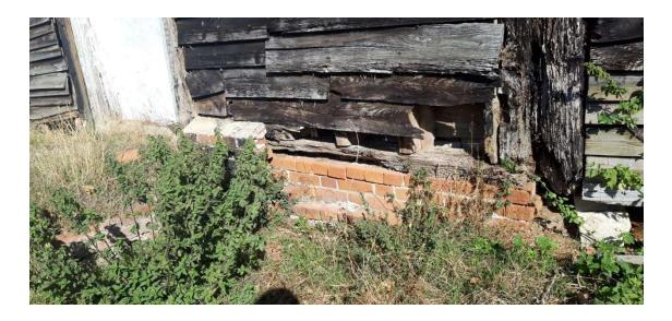
2.1.6 To the East-Central south Mistry/Cart Entrance, arrest the raking lean of the oak frame by constructing timber raking shore up the east face of the southeast post, with horizontal plate based on the solid concrete screed of the adjacent Dog Kennel Cage.
