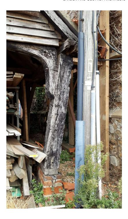
2.3.4 The principal tie beams internally are to be propped from firm ground/solid floor with Accrows where dampness and fractures/shakes have caused decay or distortion and weakened the structure.
