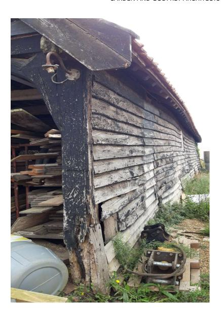
2.3.2 At south end similarly provide propping to the <u>southwest post</u>, where the sole plate and brick plinth have collapsed.
