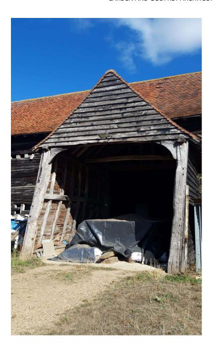
2.1.7 To the Eastern South Lean-to Boiler House, provide temporary Accrow Prop support from internal floor screed to the decayed and collapsing wall plate at west end, under eaves.
