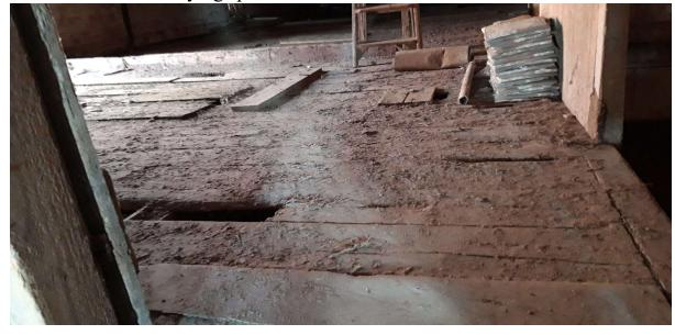
2.2.2 Prop the 1<sup>st</sup> floor where secondary N-S joists have decayed adjacent and out from the west wall above the south lobby. Acrow propping from solid floor below.
