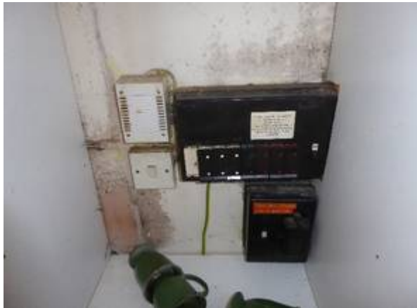
Photograph 19 – Electrical consumer unit within the base unit of the kitchen
