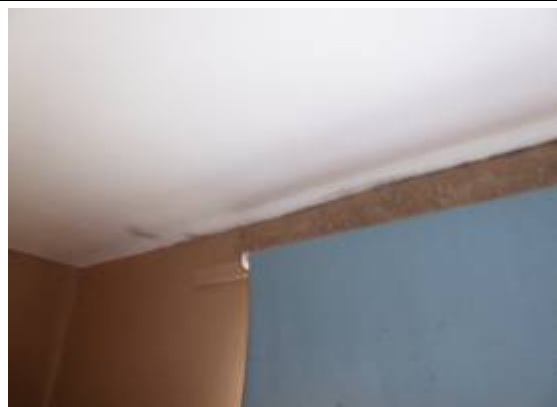
Photograph 30 – Typical image of mould to the rear bedroom ceiling
