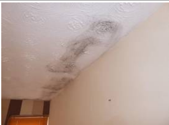
Photograph 29 – Typical image of mould growth to the rear living/dining room ceiling
