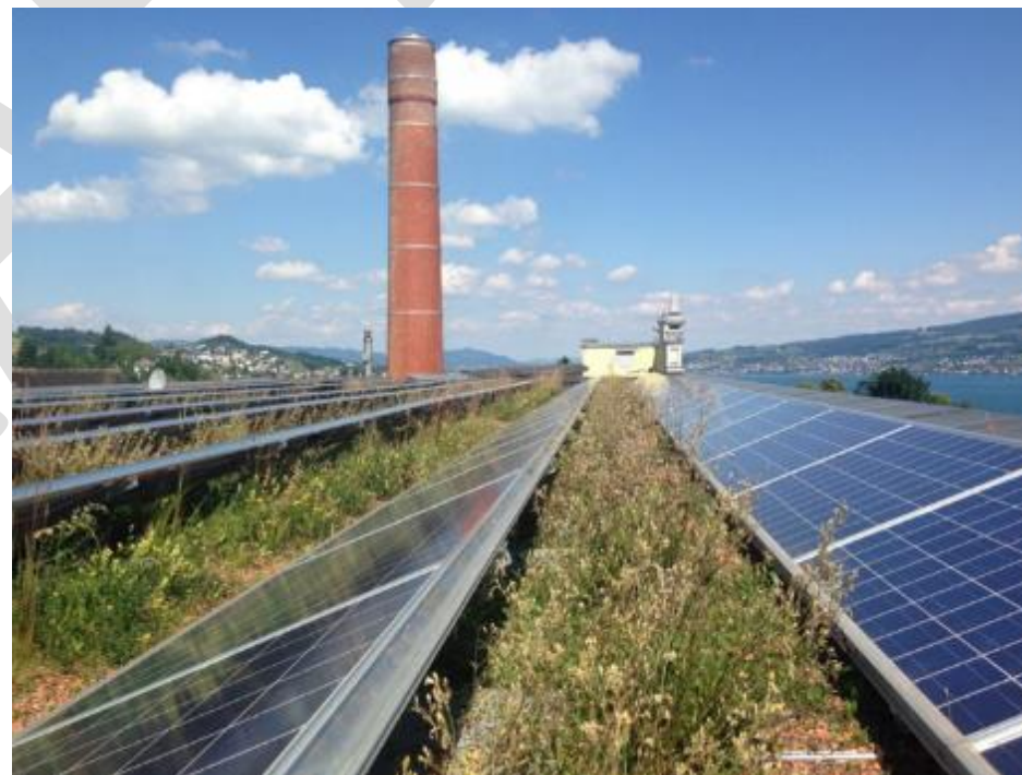
Plate 3: Biosolar roof. Credit: Green Infrastructure Consultancy
