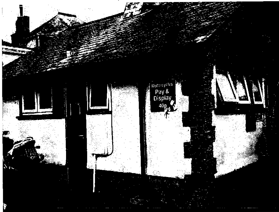
Photo 1) Showing external area to South Quay Toilets
