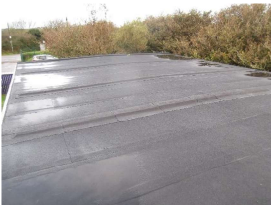
11 Modern flat bituminous felt covering
