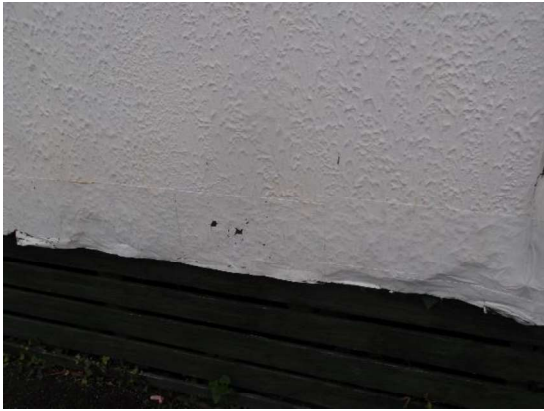
7 Panel timber – timber decay
