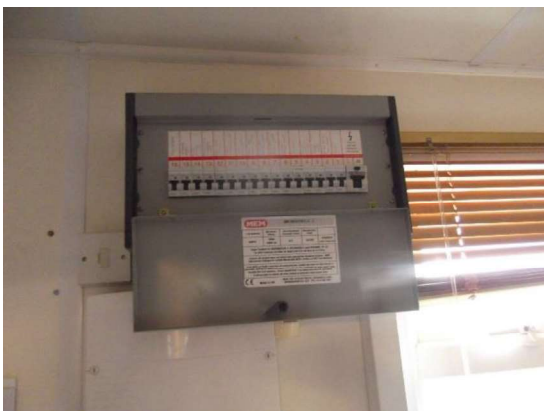
17 Consumer board – meter externally
