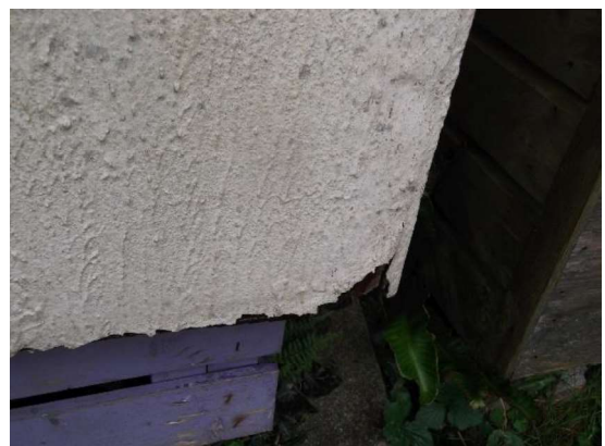
6 Panel timber – timber decay
