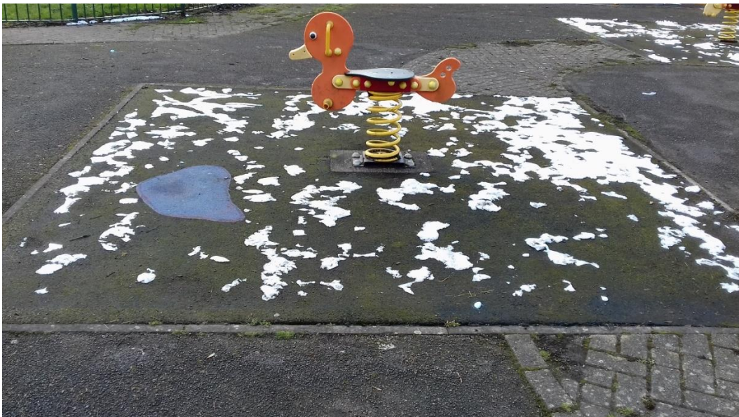
Spring flamingo – replace missing caps, wetpour strip repair
