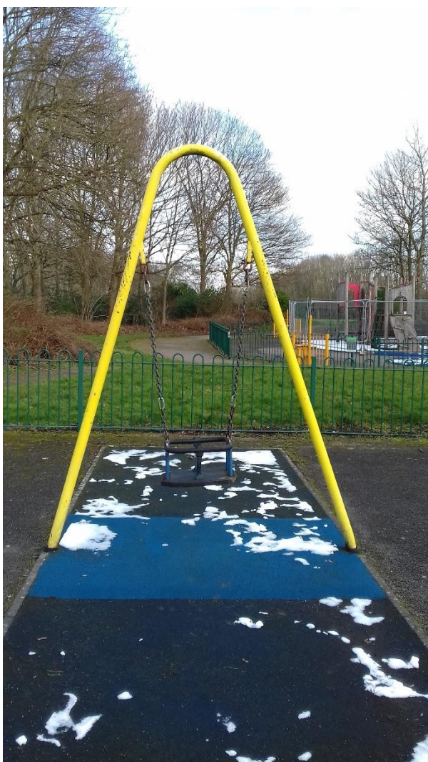
Infant swing – Dig out loose posts and re-instate, paint frame
