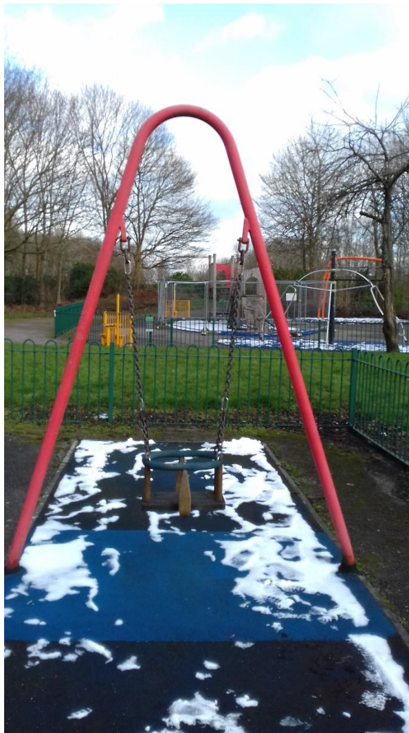
Infant swing – Dig out loose posts and re-instate, paint frame
