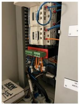
Rectifier in situ 'without frost protection', with frost protection rectifier fitted continually failing, so the work is within the wiring or windings of the anchor motor?
