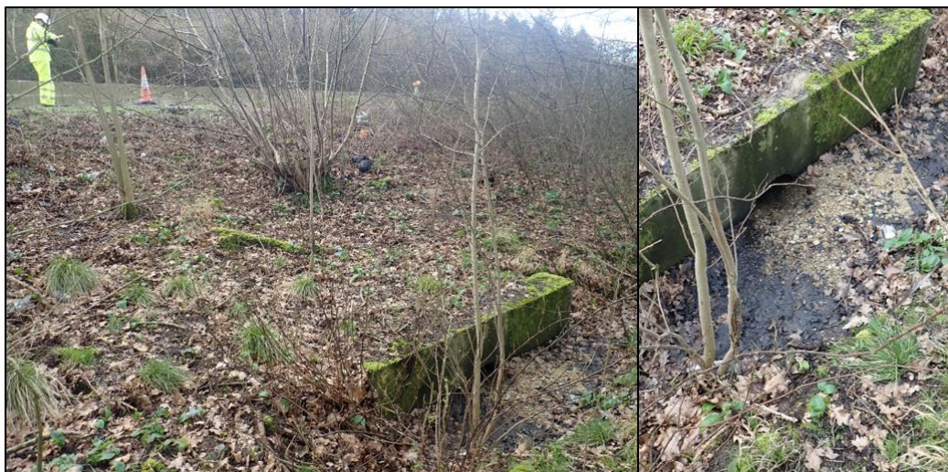
Figure 4 – View of embankment at MP125.9 EB. Debris accumulation at outfall (February 2020)
