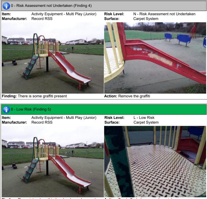
**Finding:** The paintwork on this item has been damaged or worn exposing the metal underneath which is rusting / corroding
