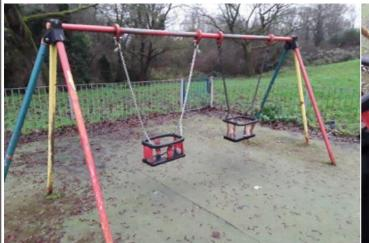
Finding: The connecting links are in excess of 8.6mm and Action: Monitor - No remedial work recommended less than 12mm and fail the requirements of BS EN 1176 Part 1; clause 4.2.13, Chains
