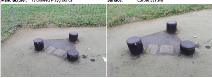
**Finding:** The step between the items is quite large and users may not be able to complete the step without touching ground, the items could therefore be considered to be within the falling space of each other, however the intention of the play activity continuity is easily apparent and foreseeable to the user
