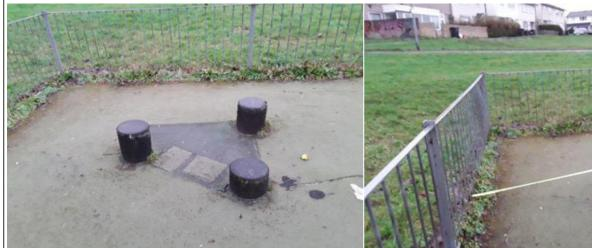
**Finding:** The fence forms a hard object within the falling space of the equipment in contravention of the requirements of BS EN 1176 Part 1
