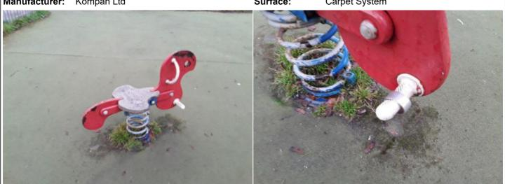
**Finding:** The end of handgrips and/or footrests have a cross **Action:** Monitor - No remedial work recommended section of less than 15cm2 and fail to meet the requirements of BS EN 1176 Part 6
