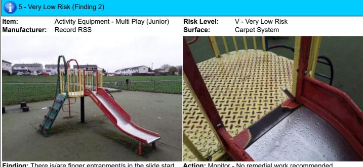
**Finding:** There is/are finger entrapment/s in the slide start **Action:** Monitor - No remedial work recommended section and the item fails to meet the requirements of BS EN 1176 Part 1 4.2.7.6 Entrapment of fingers
