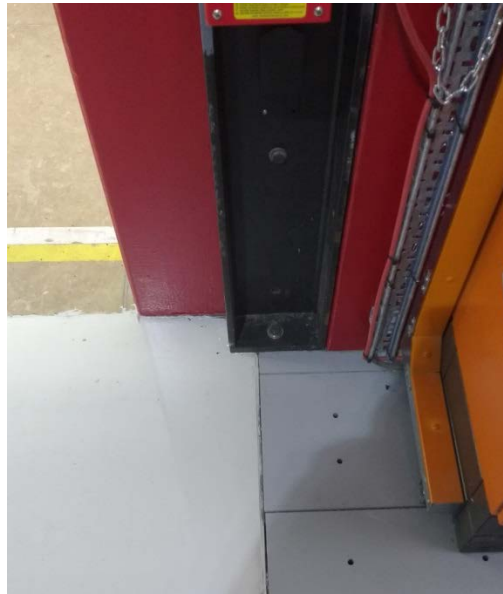
Figure 12 – Floor trench in door footprint
