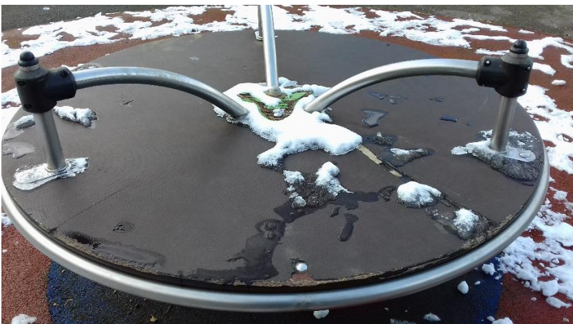
Roundabout – secure loose fixings, replace platform
