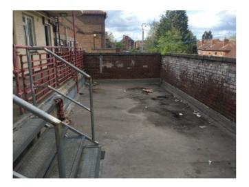
General Overview: The drying area on this block is also suffering from deck deflection leading to standing water. The water can't currently reach the chute outlets even though there is a fall on the area.
