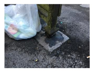
Penetrations: There are penetrations that have failed and will need to be addressed prior to any works commencing at this site.
