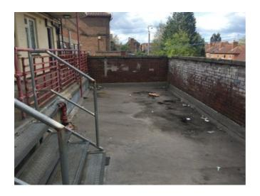
Gutters: A gutter with sufficient drainage should be formed along the entire section of the drying area prior to the installing of the tapered fall overlay.
