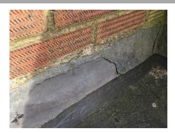
Short Term Repairs: Repairs have been carried out to the existing waterproofing. Individual repairs should be assessed for integrity and removed where necessary.
