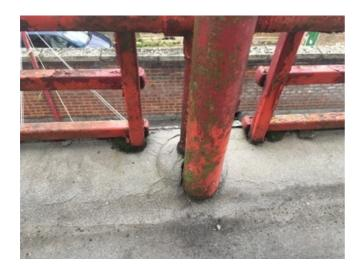
Balustrade: Remedial work will need to be carried out on the existing balustrade prior to application.
