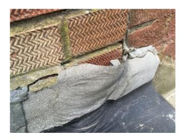
Asphalt Upstands: The asphalt has slumped on the vertical surfaces and should therefore be removed and repaired to match adjacent areas.
