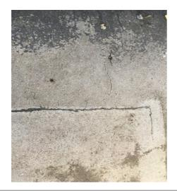
Cracking: Cracks are evident within the existing waterproofing. The cause of the cracks may require further investigation and all necessary action taken to eliminate reoccurrence.
