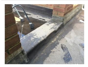
General Overview: The small drying area on this section of the flats is suffering from major deck deflection, meaning water is ponding in the middle and not able to reach the outlet in the corner.
