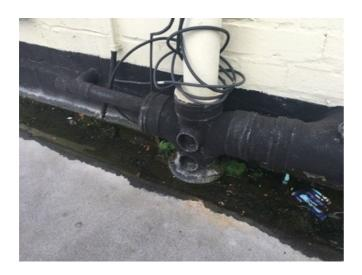
Penetrations: Remedial work will need to be carried out to all penetrations prior to works starting as currently they are not in a fit state to be coated with the new system.
