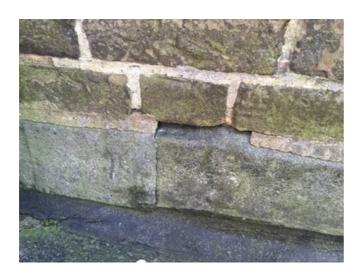
Upstands - Brickwork: The existing brickwork chase has been patch repaired using a felt material. This has now failed and ripped in several places. There are areas where the chase mortar has blown allowing moisture to enter the internal structure. This is to be repaired prior to coating.
