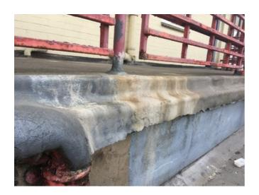
Upstand abutment detail - Plyboard: The interface between the low level walkway and the drying area needs to be remedied as part of these works. This is to include the knocking back of the original asphalt, redirection or removal of the wrought iron pipework and a ply-board face being installed.
