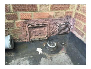
Outlets: Remedial work may be required prior to the application of the waterproofing system involving cutting back, levelling and removing obstructions to allow efficient drainage.
