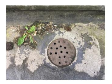
Outlets: Remedial work required prior to the application of the waterproofing system involving cutting back, levelling and removing obstructions to allow efficient drainage.
