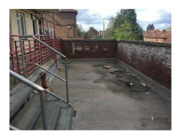
Asphalt Condition: The existing asphalt has failed and is no longer an effective waterproofing although it is considered suitable for overlay.
