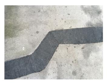
Asphalt Condition: The existing asphalt has failed and is no longer an effective waterproofing although it is considered suitable for overlay.
