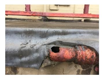
Outlets: Remedial work is required prior to the application of the waterproofing system involving cutting back, levelling and removing obstructions to allow efficient drainage.
