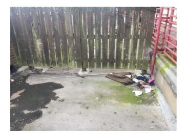
Ponding: Standing water is an issue in places, increasing the likelihood of water ingress via defects in the existing waterproofing.
