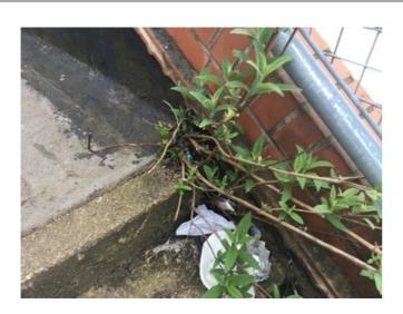
Perimeters - Vegetation Growth: There are several areas where trees and plants have taken root in the brickwork due to poor detailing and failure of the waterproofing system. All to be removed and areas treated as per manufacturers requirements .
