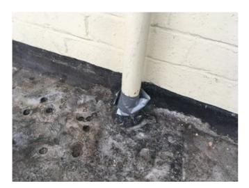
Penetrations: Remedial work will need to be carried out to all penetrations prior to works starting as currently they are not in a fit state to be coated with the new system.
