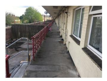
General Overview: The waterproofing on these walkways is in a similarly poor state to the other areas. There are several areas where old cracks have been patch repaired and pipework has been also patched.
