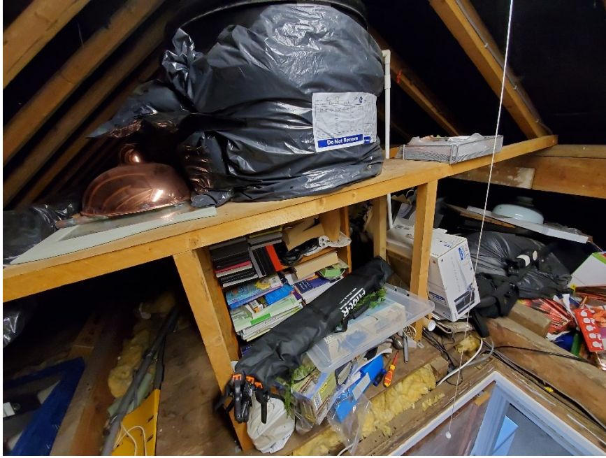
Figure 13 – Water tank and timber structure
