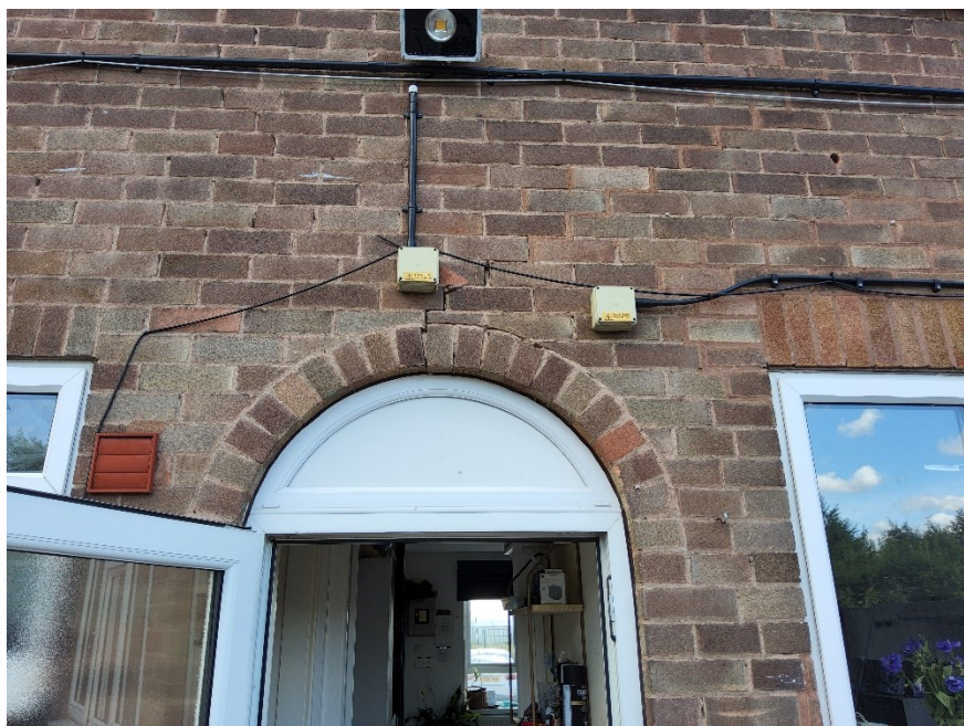
Figure 10 – Cracked arch
