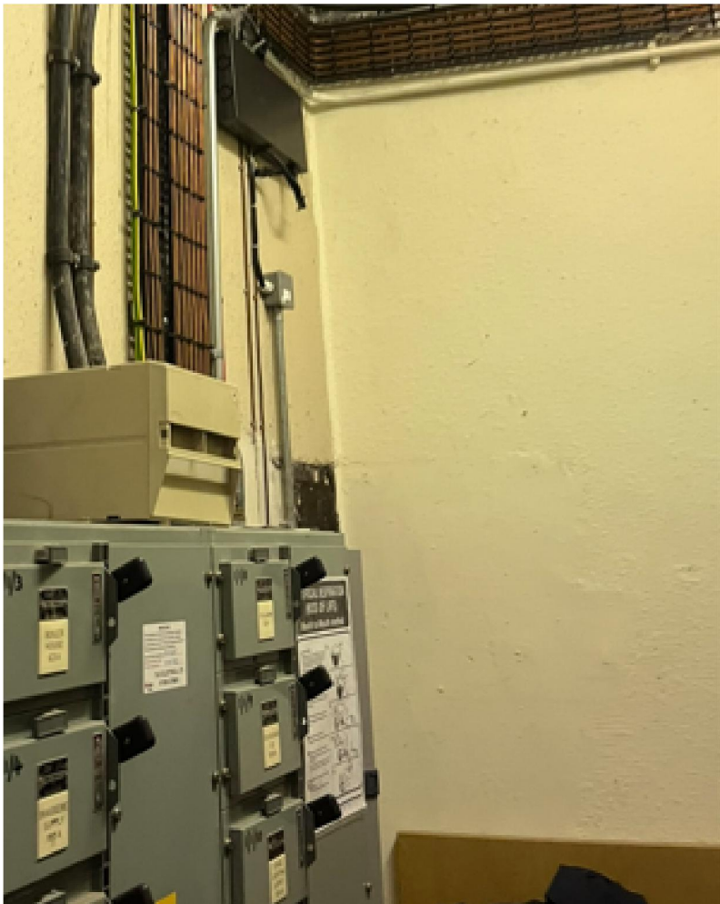
PROPOSED VACANT WALL SPACE ADJACENT TO ELECTRICAL SWITCHGEAR IS TO HOUSE NEW PV INVERTER
