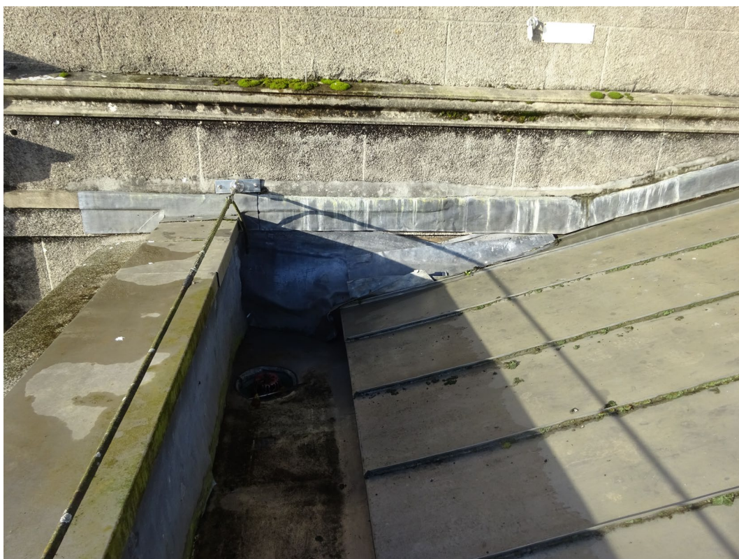
12. Displaced leadwork to S6 west
