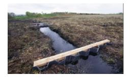
A cross-section of the topography in this part of the floodplain, provided by Peter Stone, suggests that the metal piling dams in this ravine should be at least 6m wide x 2m (1m above surface + up to 1m below surface) in dimension. The piling should be driven down into the surrounding peat, so that the top is flush with the surrounding floodplain (pictured above).
