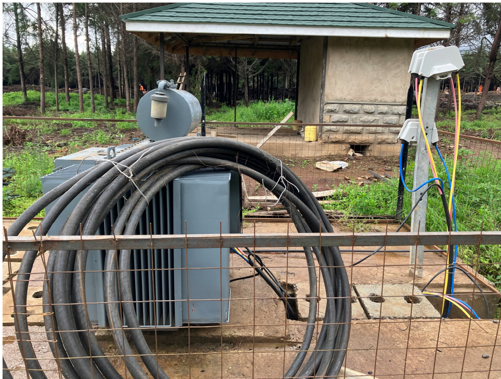
Figure V11.1. Existing Transformer, LV Cut-Outs and KDF's new LV switchboard Building.
