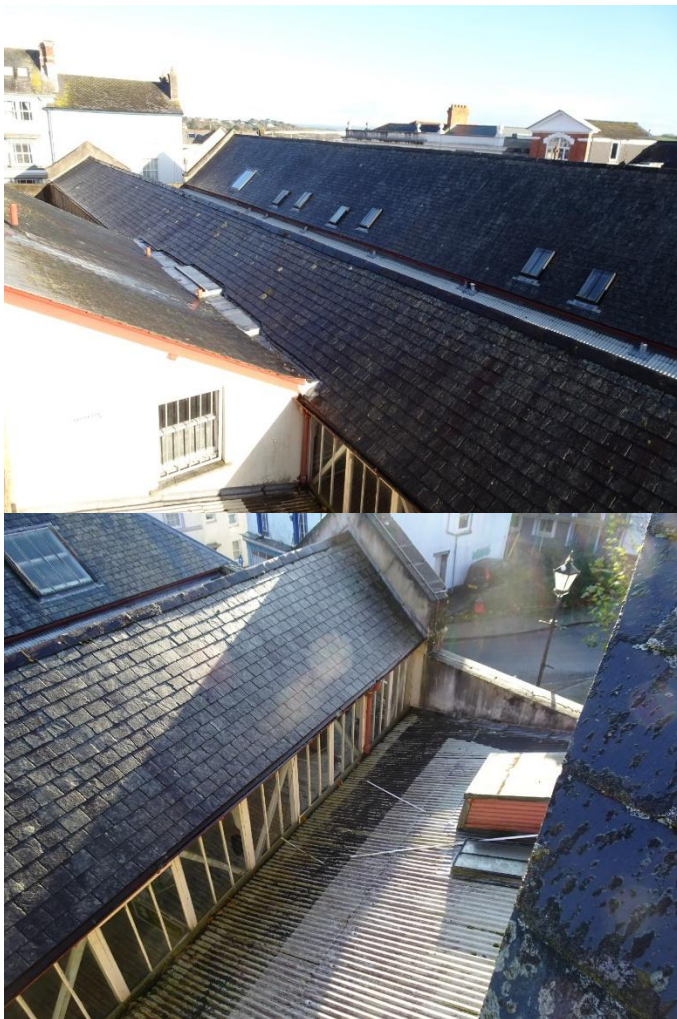
2. Butcher's Row: Combination of slate and corrugated sheet roofing.
