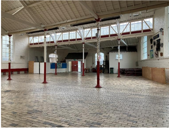
3. Market Hall: Interior looking North West. Sarking boards to underside of slate roof.
