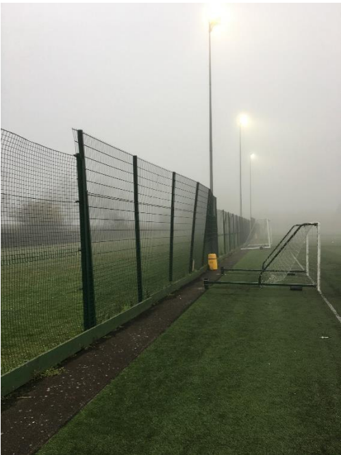
(8). Fence posts need resetting as all are loose and leaning towards the pitch.
