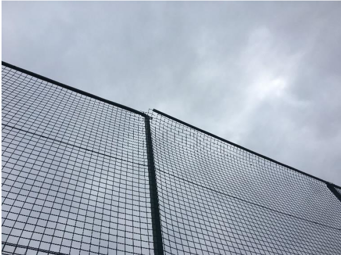
(11). Top rail bar loose and needs reattaching.
