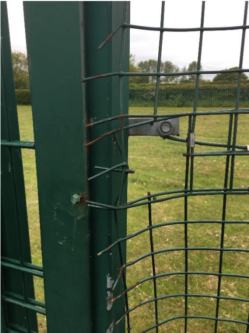
(9) Mesh panel loose from clamp rail.
