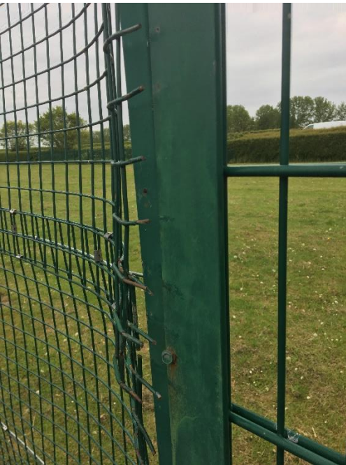
(7) Mesh panel loose from clamp rail.
