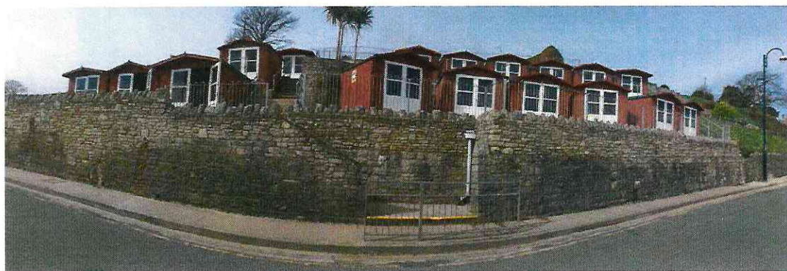
View of holiday chalets, looking west from Shore Road.
