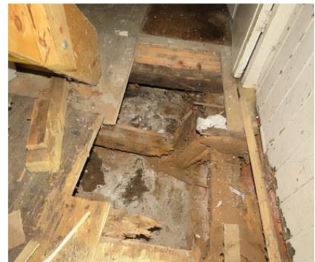
Timber decay and beetle activity to rotten floor beneath stairs.
