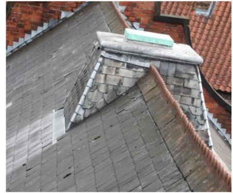
Cupola flashings slipped and missing. Cupola capped with copper.
