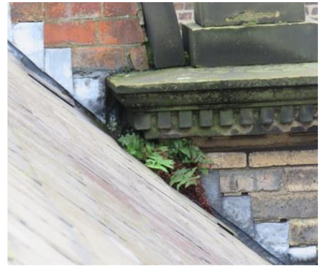
Plant growth in flashings behind gables.
