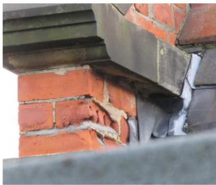
Spalled bricks/poor pointing behind Morton Lane entrance parapet.
