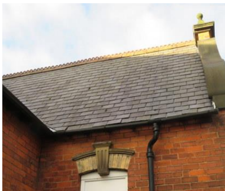
Open joints to ridges to entrance roof.
