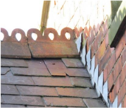
Poor flashings to gables. Slipped/missing slate.
