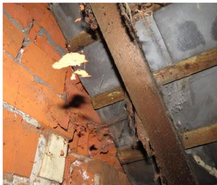
Spalled bricks to Wilbert lane gable.
