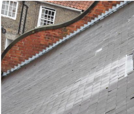
Missing/slipped slates to all slopes.
