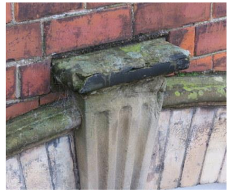
Stone details above windows spalling/cracked.
