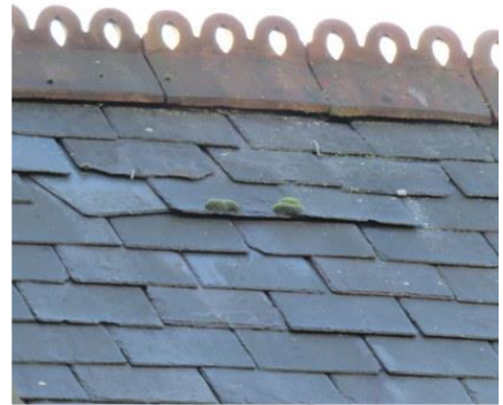
Pointing generally to ridge missing. Tingles in place in various locations.
