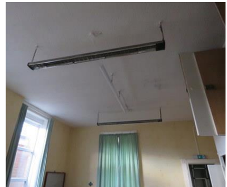
Heating via wall and ceiling mounted electric radiant heaters.
