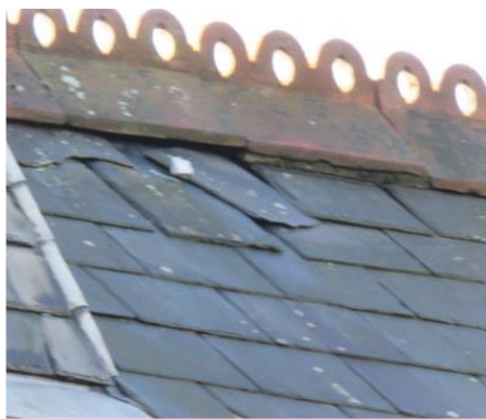
Slipped/missing slates to Morton Lane slope.
