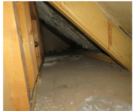
Condensation mold growth to plaster lath in eaves voids.
