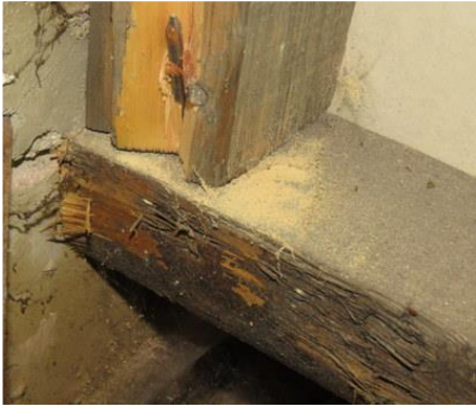
Frass evident to the rear slope eaves construction.
