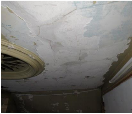
Plaster lath ceilings in top floor blown/effected by condensations.
