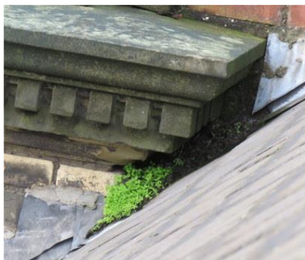
Plant growth in flashings behind gables.
