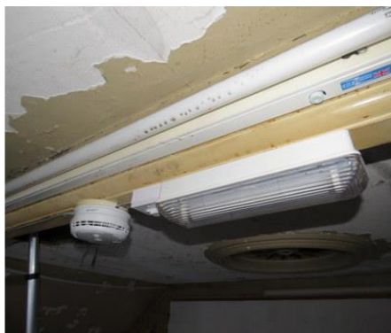
Smoke detection in first floor. Emergency lighting throughout.
