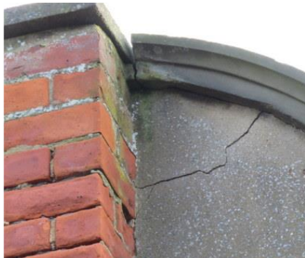
Cracking to high level render to chimney.
