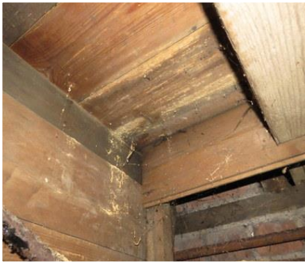
Beetle activity to underside of floor boards.
