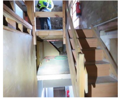
Balastrade not compliant with current regulations.
