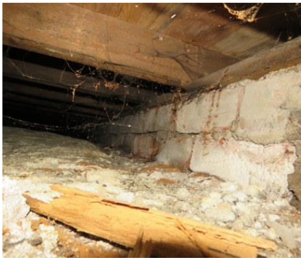
Mycellium evident below hall floor.
