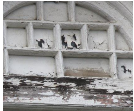
Decay to remaining timber windows.
