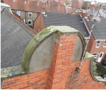
Chimney has been capped.
