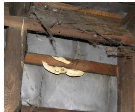
Fruiting body on timber lats beneath cupola.
