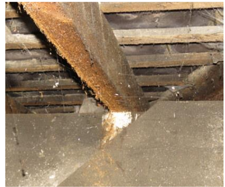
Wet purlin and rafter adjacent to Morton Lane entrance roof.
