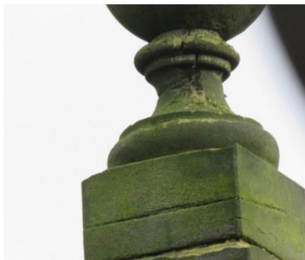
Cracking to stone support on finial on Morton lane gable.
