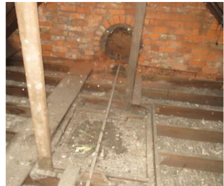
Plaster lath evident. Mech fitted behind ceiling vents.
