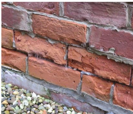
Low level brickwork spalled and pointing poor.
