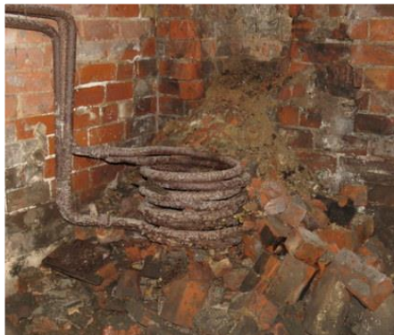
Redundant heating coil to perimeter underfloor heating.
