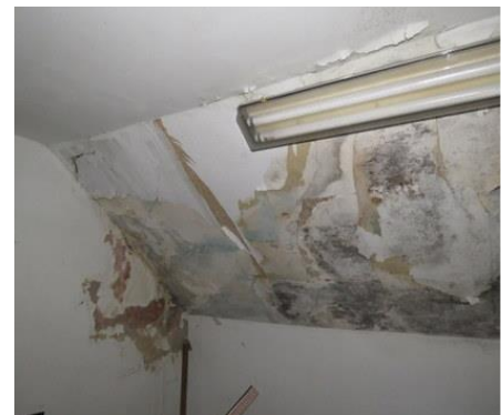
Plaster lath ceilings in top floor blown/effected by condensation.
