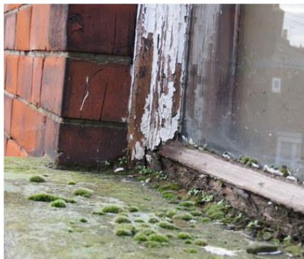
Decay to remaining timber windows.
