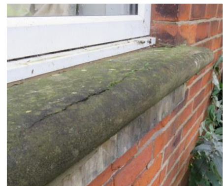
Stone cills cracking in various locations.
