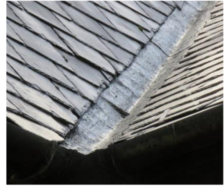
Liquid repair to valley gutter.
