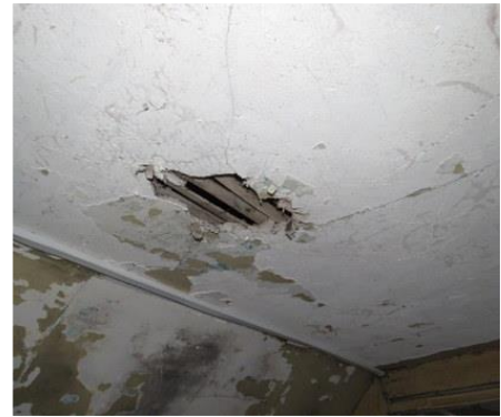
Delaminated sections of plaster lath throughout first floor areas.
