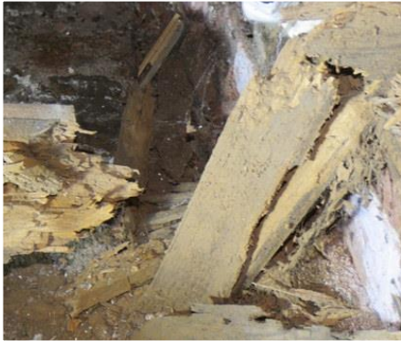
Timber decay to stairs floor void.
