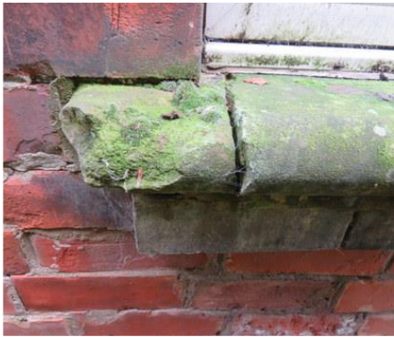
Damaged/cracked stone cills to a number of windows.
