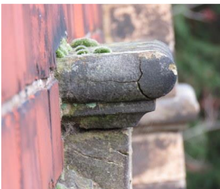
Stone details above windows spalling/cracked.
