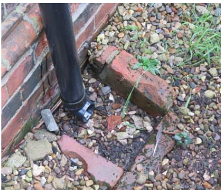
Soak aways to some rainwater outlets.
