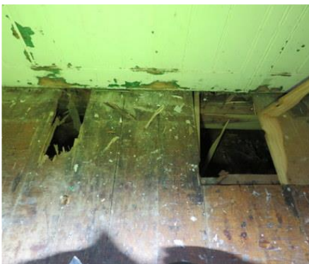
Rot to floor structure in main hall.
