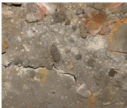
Floor beneath void has a degrading surface.
