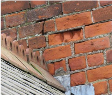
Spalled bricks, poor pointing to rear of Wilbert lane gable.
