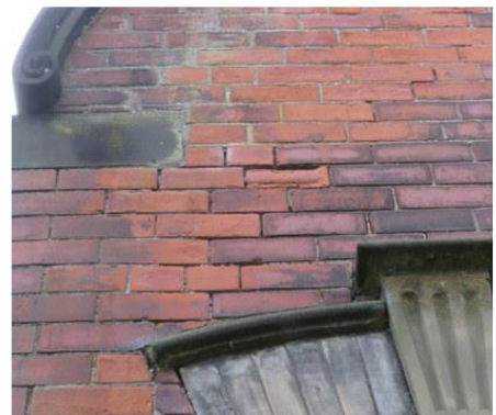
Stepped cracking above Morton Lane entrance.
