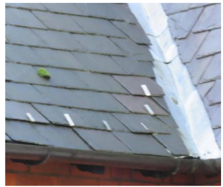
Tingles evident to entrance roof.
