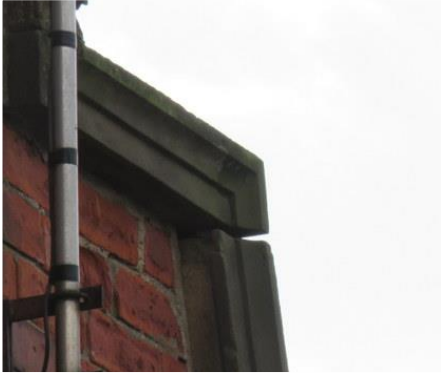
Open joints to gable parapet capping stones.
