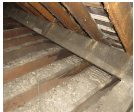
A number of rafters and joist were wet at the time of inspection.
