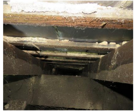
Void between roof and eaves parging loose and missing in various locations.
