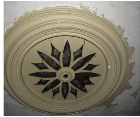
Damage to ceiling vents.
