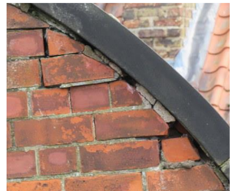
Loose brickwork and open joints to gable beneath capping stones.
