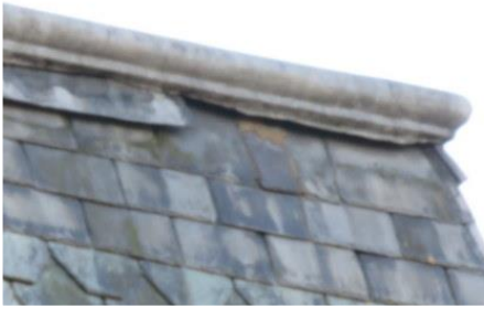
Missing flashing to cupola.
