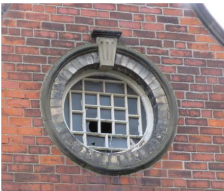
Broken glass to round window above Morton Lane entrance.
