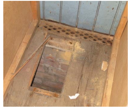
Frass evident to floor beneath cupboard in kitchen.
