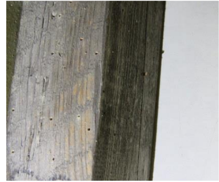
Beetle flight holes in timbers to rear roof slope eaves.
