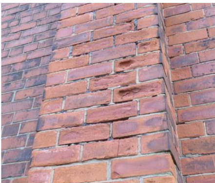
Spalled bricks and open joints to chimney.
