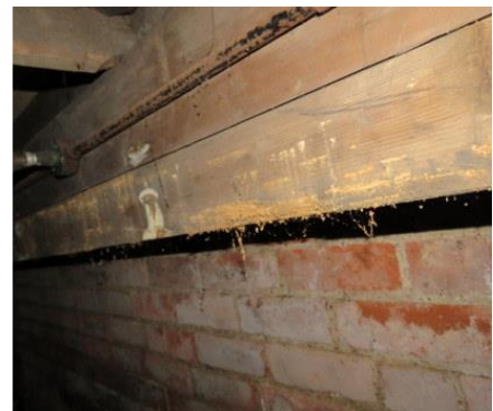
Beetle activity to floor joists beneath main reception room.
