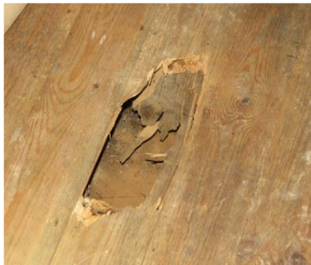
Beetle activity to floor void at corner of Wilbert and Morton lane.
