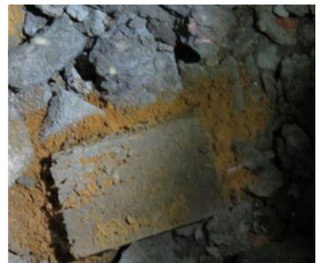
Beetle activity in floor void.
