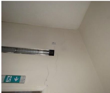
Cracking to wall above entrance into hall.
