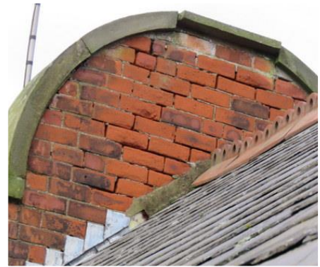
Poor pointing to rear of Morton Lane gable. Section of flashing replaced with sand cement.
