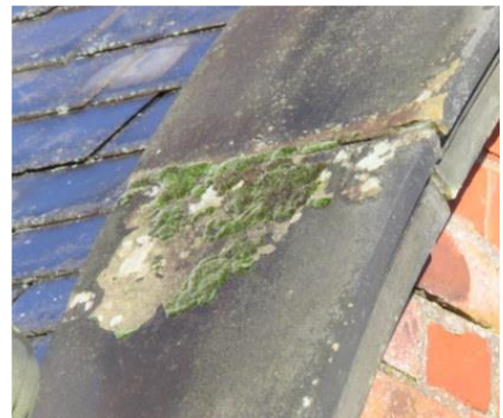
Stone starting to spall to parapet cappings.
