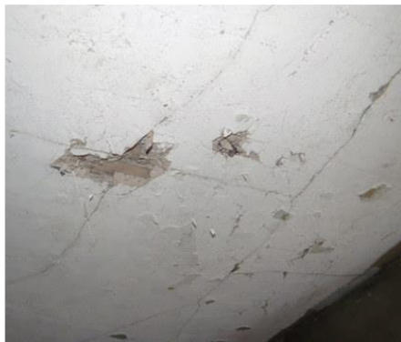
Delaminated sections of plaster lath throughout first floor areas.
