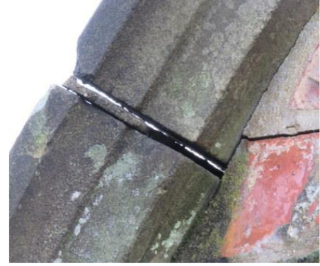
Open joints to gable parapet capping stones.
