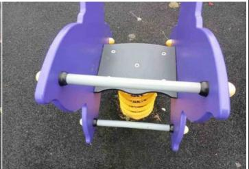
**Finding:** The Handgrips/Footrests rotate and may cause an **Action:** Secure Handgrips/Footrests to prevent rotation. unexpected movement for the user
