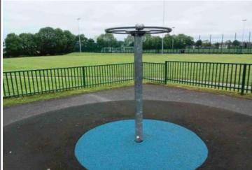
**Finding:** There is/are finger entrapment/s in the handgrip and the item fails to meet the requirements of BS EN 1176 Part 1 4.2.7.6 Entrapment of fingers
