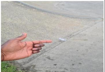
**Finding:** Joints between the riding / rolling surfaces shall not **Action:** Take corrective action to ensure that the gaps be greater than 5mm in contravention of the requirements of between the joints do not exceed 5mm BS EN 14974 – 6.2.4
