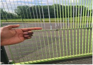
**Finding:** The weld(s) on this item have failed leaving sharp **Action:** Repair item edges
