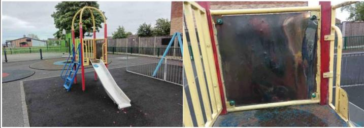
Finding: There is some evidence of fire damage to the item Action: Monitor for any further deterioration and repair as required
