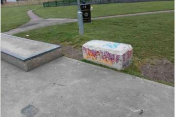
**Finding:** The item has insufficient safety zone allowed as required by BS EN 14974 - 6.4. This should equal at least 2.0 metres on this item
