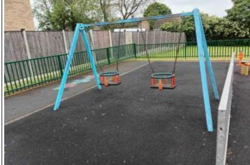
**Finding:** The chain links are worn excessively and require renewing
