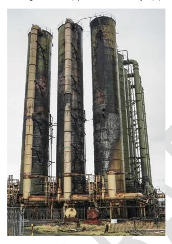
In addition to the dismantling/demolition of the ammonia washers the main works includes;
