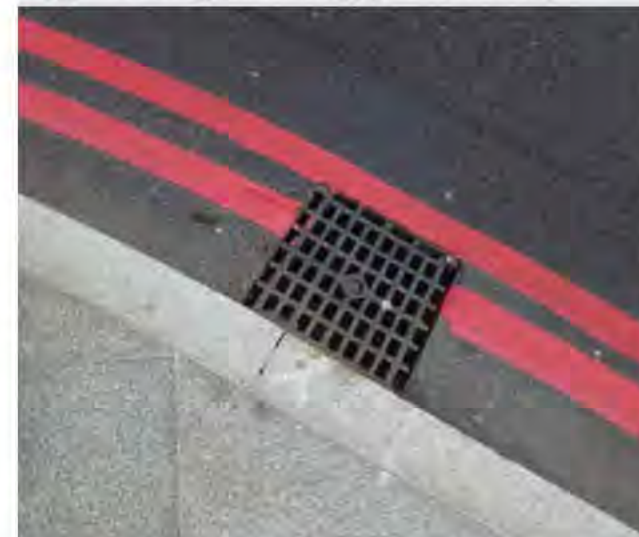
Figure 275: Cycle friendly grate on TLRN
