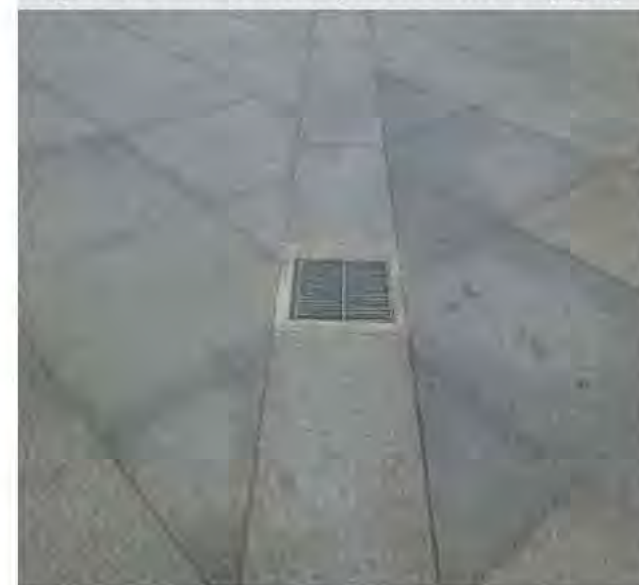
Figure 276: Channel and pedestrian friendly gully
