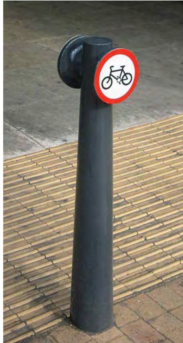
Figure 247: Integrated bollard mounted cycle signage
