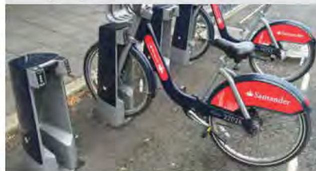
Figure 222: An inset cycle hire docking point on a steel plate
