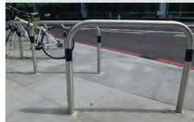
Figure 217: Cycle stands must have a contrasting visibility band
