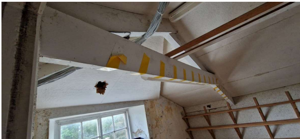
Figure 32: Photograph of 'A-frame' or 'raised collar tied' trusses to north wing
