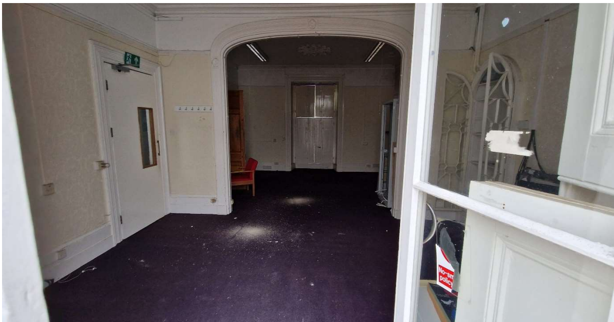
Figure 26: Photograph showing typical ground floor room
