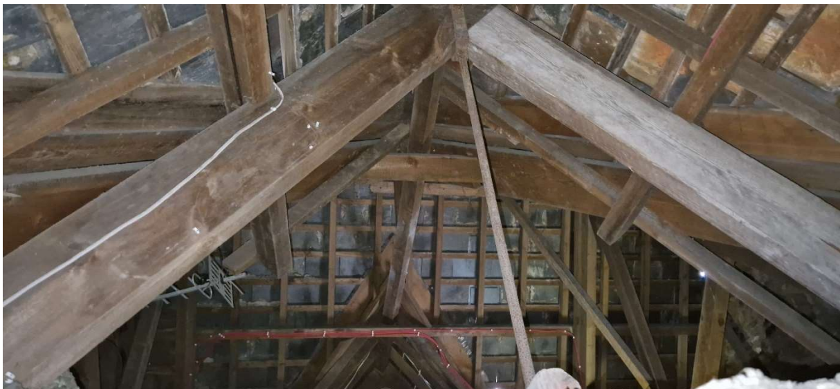
Figure 11: Photograph of Area R7a in roof space above ceiling level
