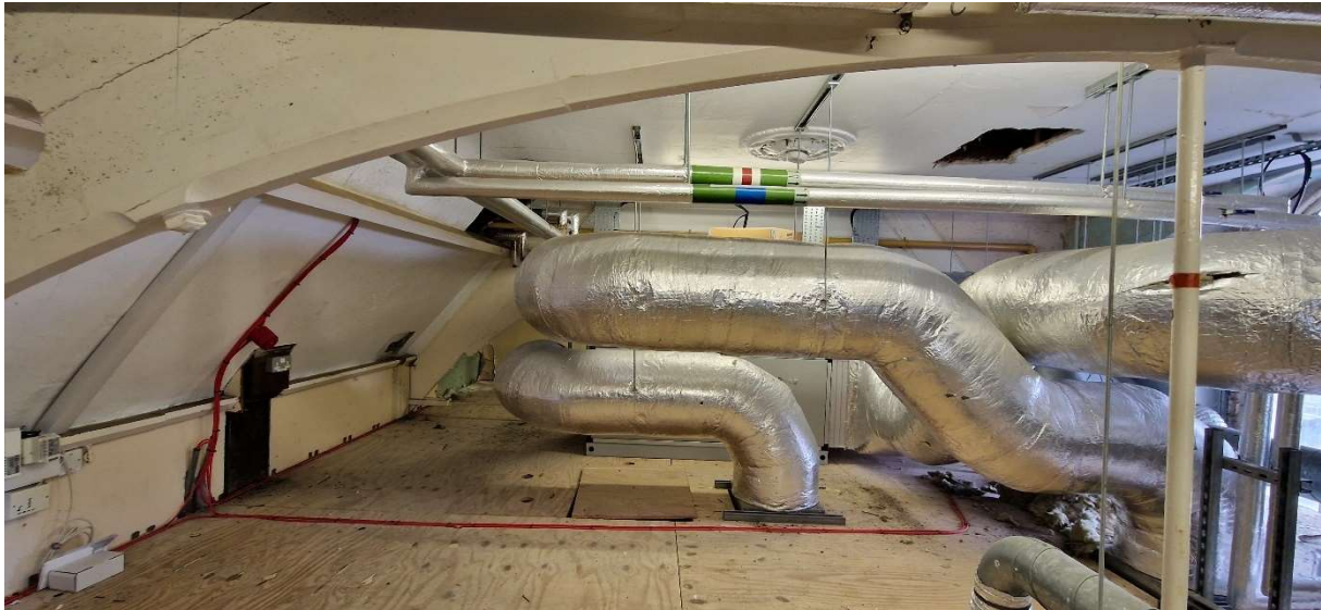
Figure 10: Photograph in Area R7a showing plant deck
