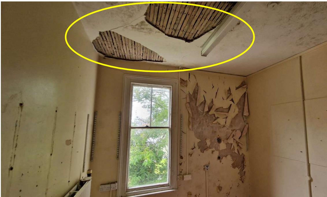
Figure 28: Photograph taken at first floor level showing lathe and plaster ceiling
