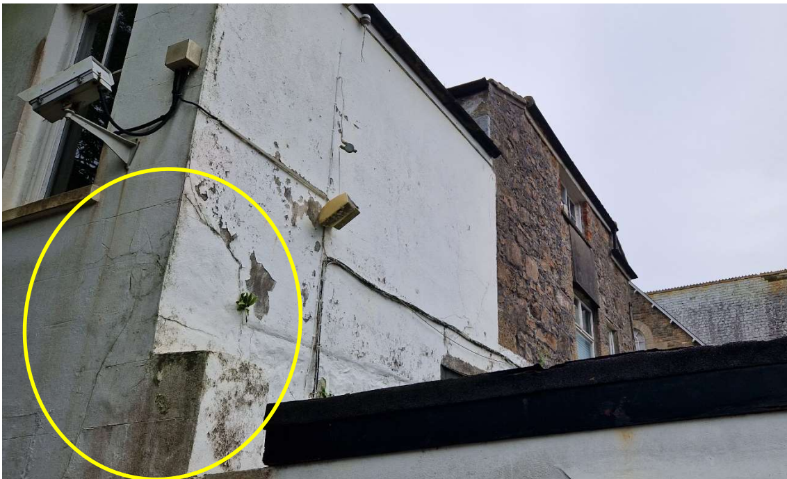
Figure 39: Photograph showing west elevation of White House
