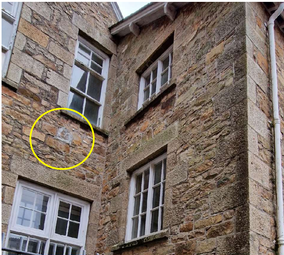
Figure 13: Photograph showing masonry repair with cementitious mortar
