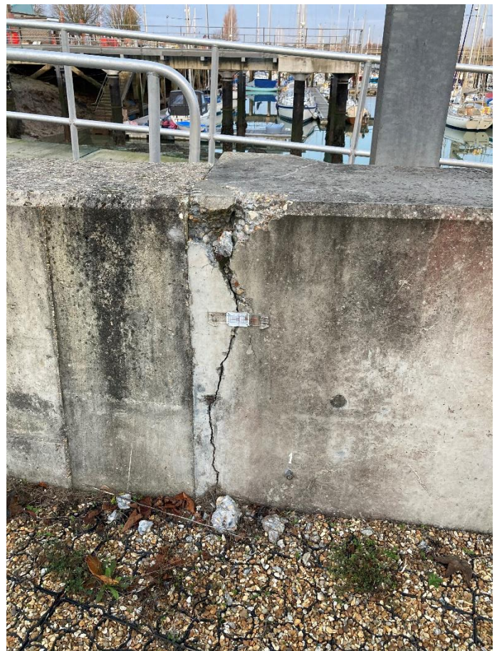
Transition joint cofferdam to ramp (crack)
