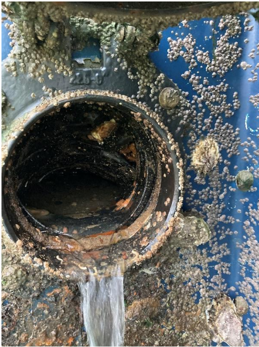
Drainage point 4 (collapsing breaking away)
