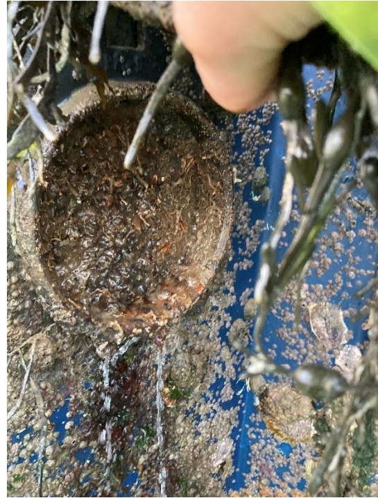
Drainage point 5 (collapsed and blocked)
