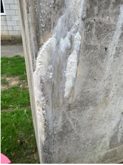
Figure 3: Foundation block seepage
