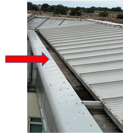
Fig 16 Debris to channel
