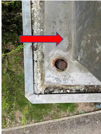
Figure 43: Light pitting to baseplate
