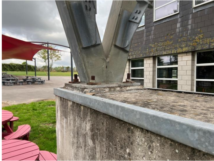
Figure 21 – Staining to foundation block & corrosion to pier
