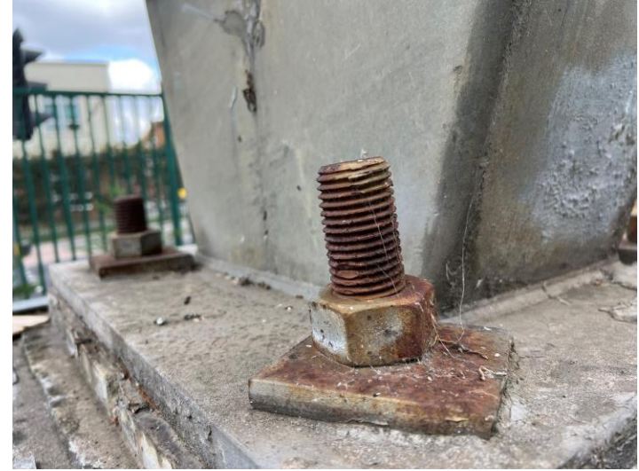
Figure 22 – Corrosion to HD bolt and washer
