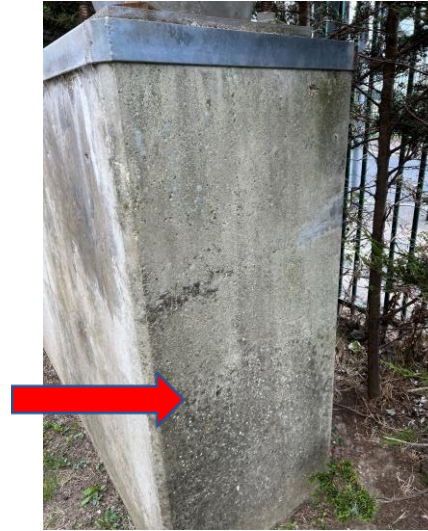
Figure 31: Staining to West block
