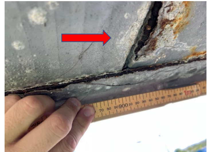
Fig 2 Heavy corrosion
