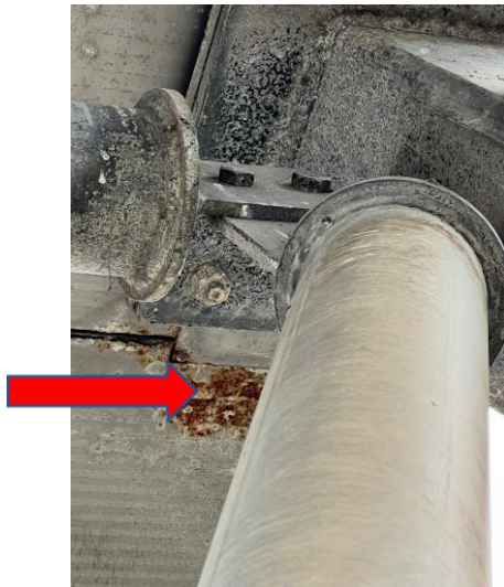
Fig 13: Light corrosion
