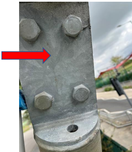
Fig 25: Strut junction light damage
