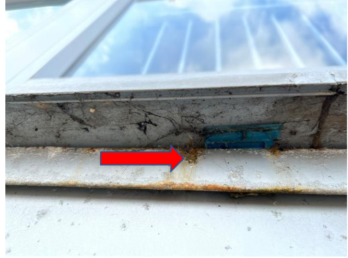
Fig 30 Heavy corrosion
