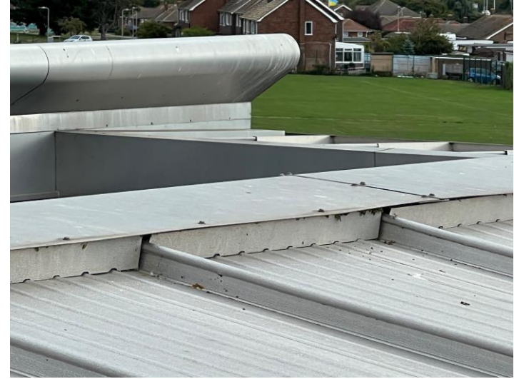
Fig 22 Gaps to infill panels
