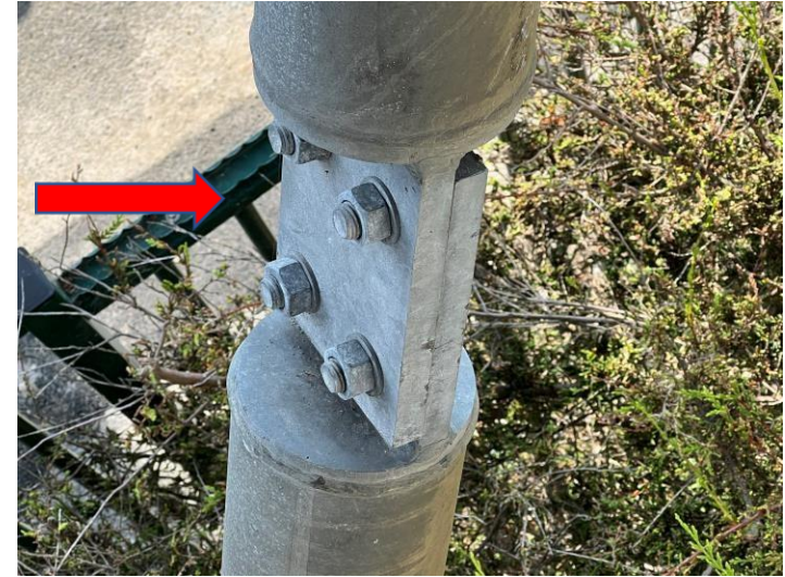
Fig 16 Brace mid connection
