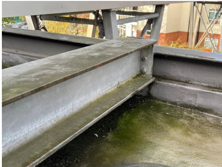
Image 15: Lack of edge protection
