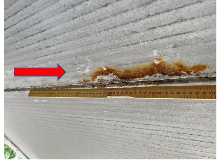
Fig 24 Heavy corrosion
