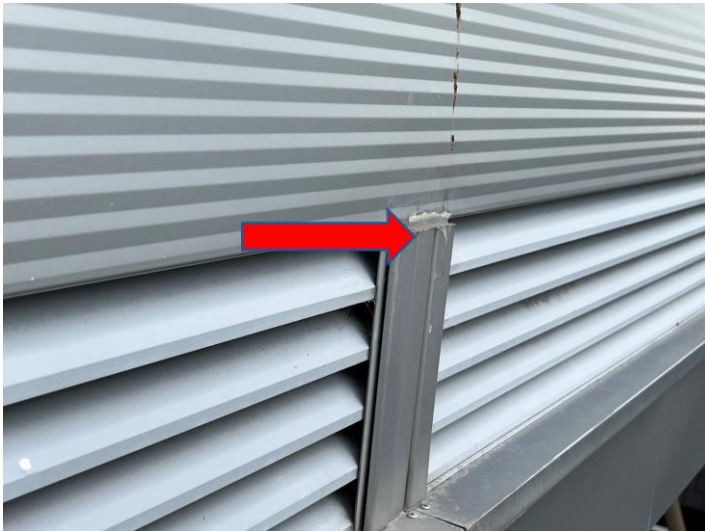
Fig 28 Light pitting to cover fillet
