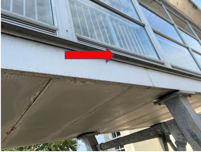
Fig 9 Moderate corrosion
