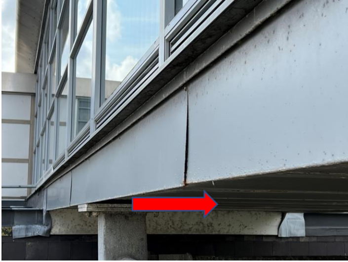
Fig 33 Corrosion at all panel junctions
