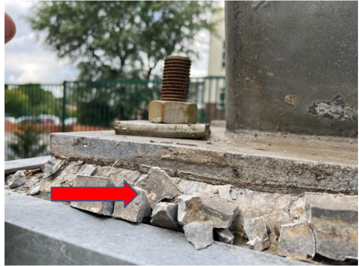
Figure 8: Degradation to grout
