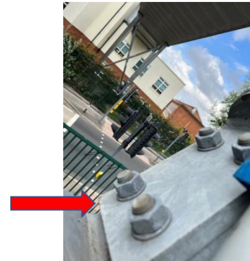
Fig 14: Corrosion to struts
