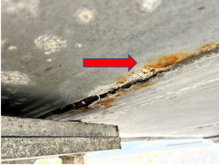
Fig 29 Heavy corrosion
