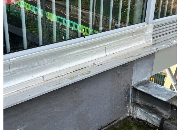
Image 6: Flash band to external cladding
