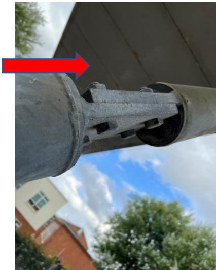
Fig 17: Light corrosion
