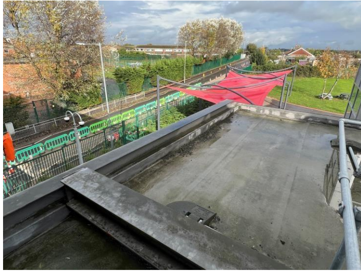
Image 15: Lack of edge protection
