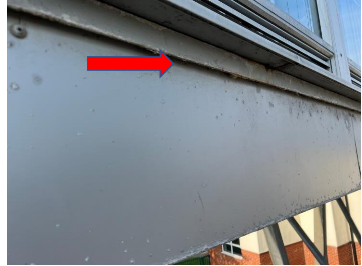
Fig 4 Moderate corrosion
