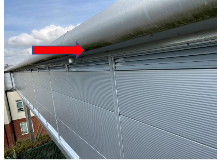
Fig 12 Moss to soffit roll
