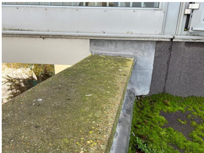
Figure 1: Lack of edge protection
