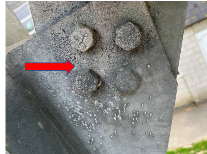
Fig 6: Light corrosion
