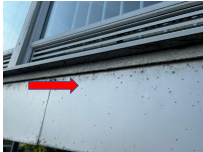
Fig 6 Moderate corrosion
