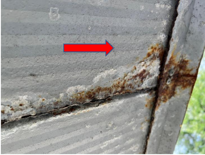
Fig 5 Delamination
