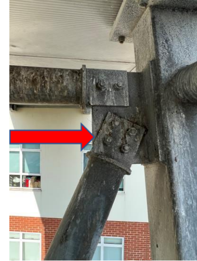
Fig 10 Moderate corrosion
