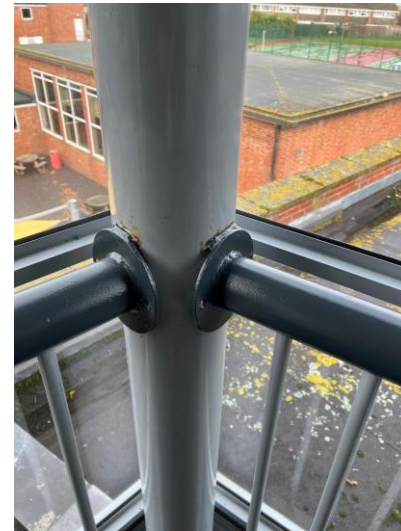
Figure 15: Upright mid section light corrosion
