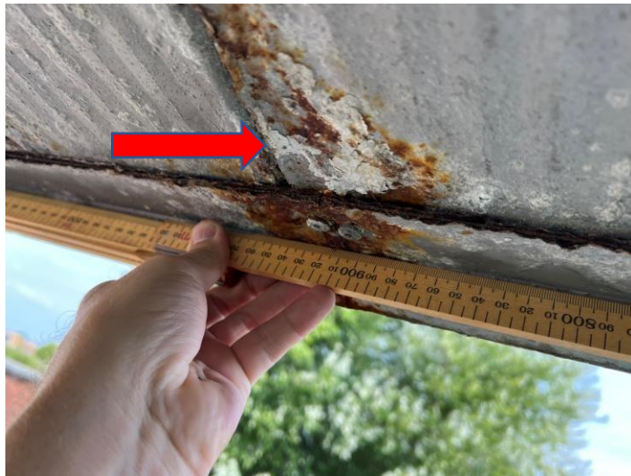
Fig 1 Moderate corrosion
