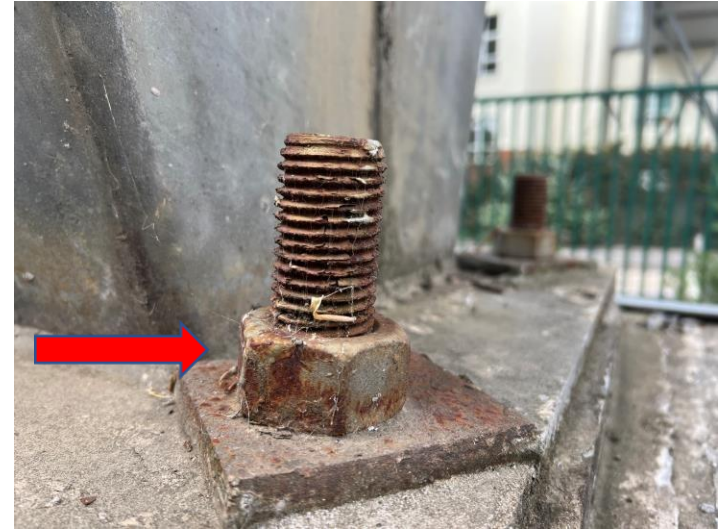
Figure 18: Moderate corrosion to HD bolt & packer
