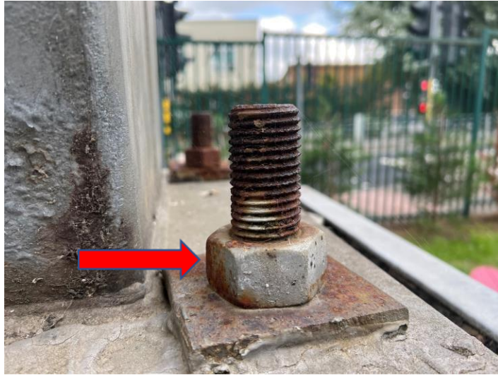
Figure 25: Moderate corrosion
