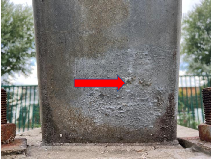
Figure 13 – Pitting damage & corrosion
