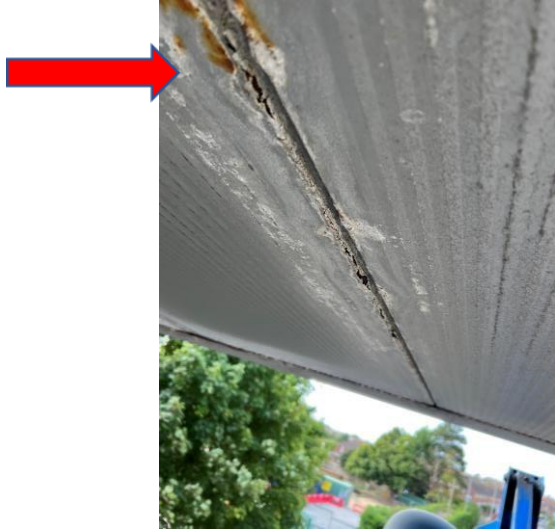
Fig 21 Heavy corrosion & delamination
