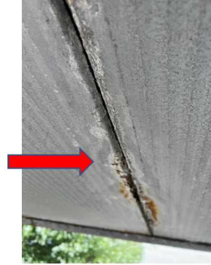
Fig 18 Heavy corrosion
