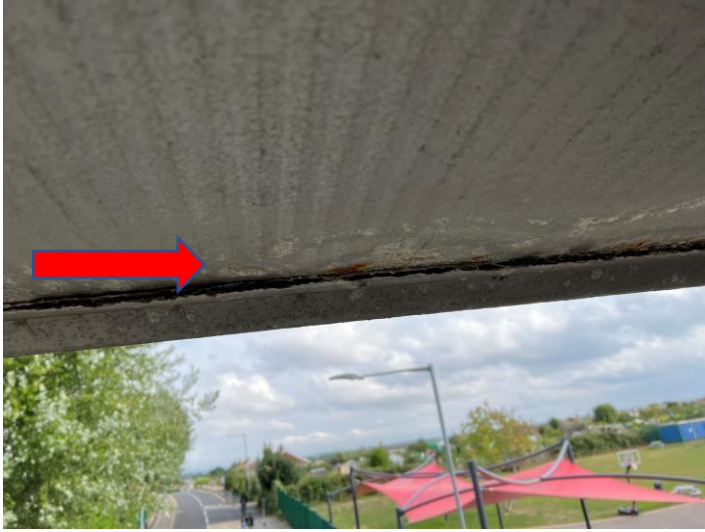
Fig 17 Moderate corrosion
