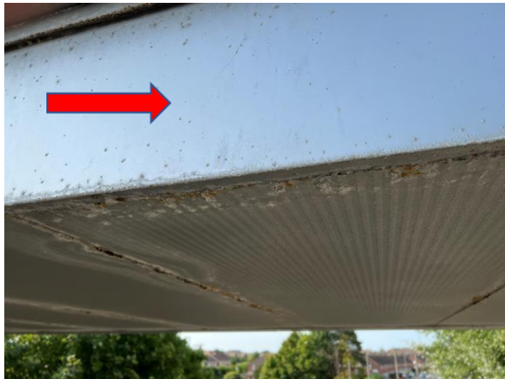
Fig 1 Light corrosion
