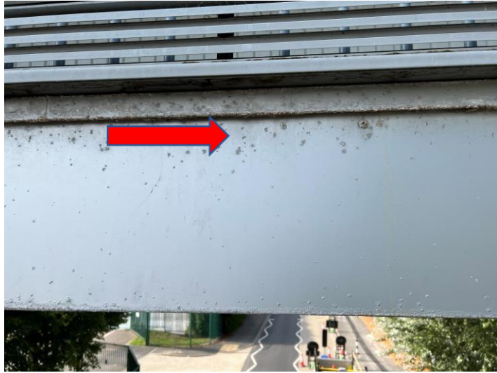
Fig 1 Light corrosion
