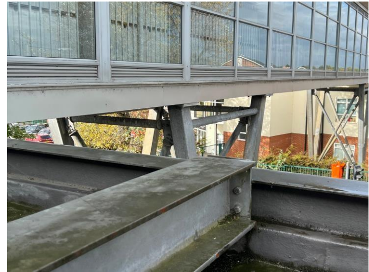
Image 16: Lack of edge protection
