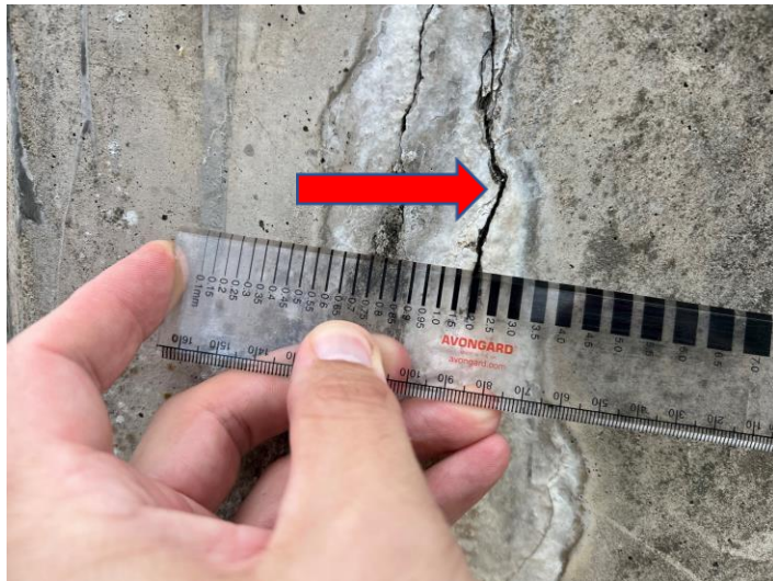
Figure 25: Moderate corrosion
