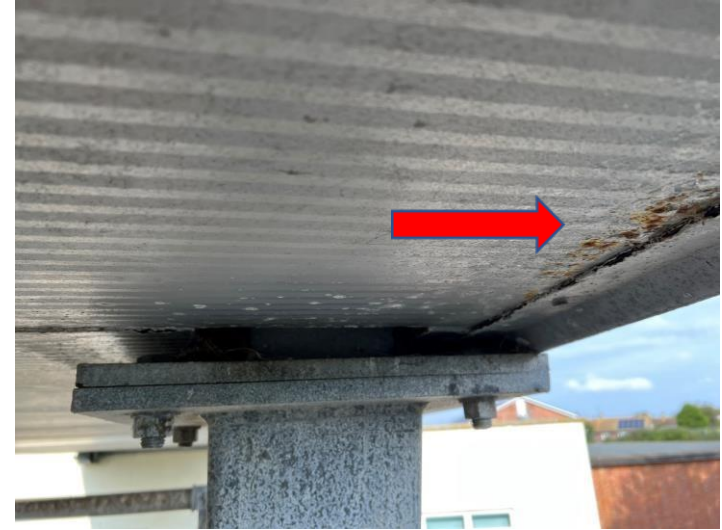
Fig 8 Light corrosion & pitting
