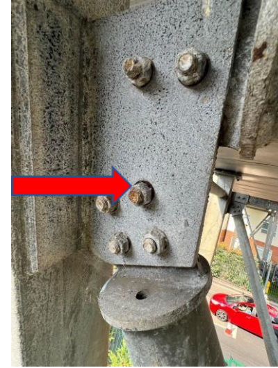
Fig 36 Moderate corrosion & washer corrosion
