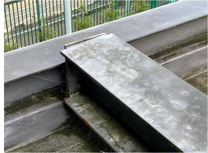
Image 14: Light corrosion
