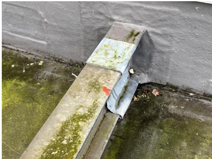
Image 9: Flash band to external cladding
