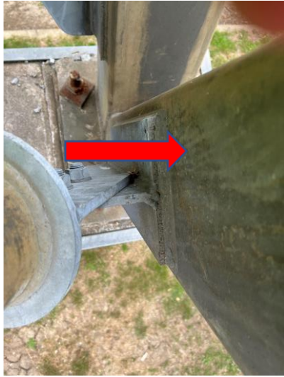
Fig 19: Light corrosion
