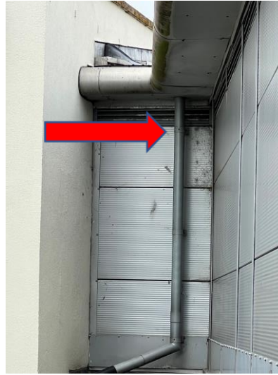
Fig 27 Rain water outlet
