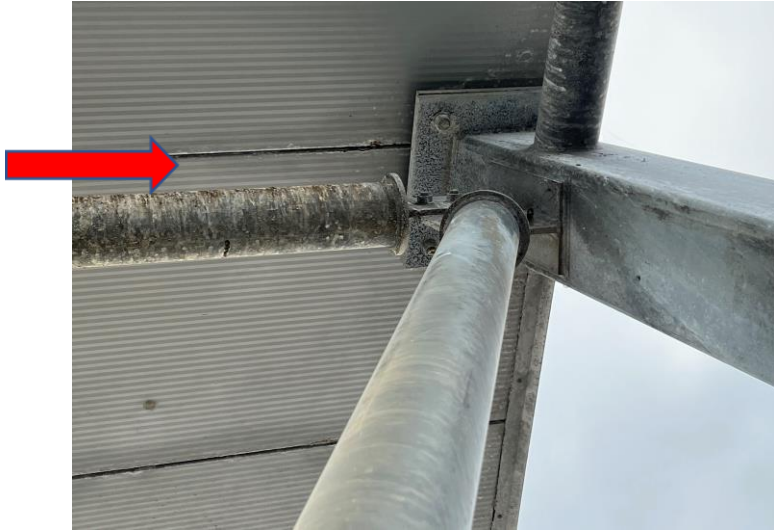
Fig 37: Moderate corrosion & pitting & pigeon guano
