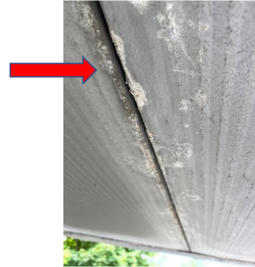
Fig 26 Delamination
