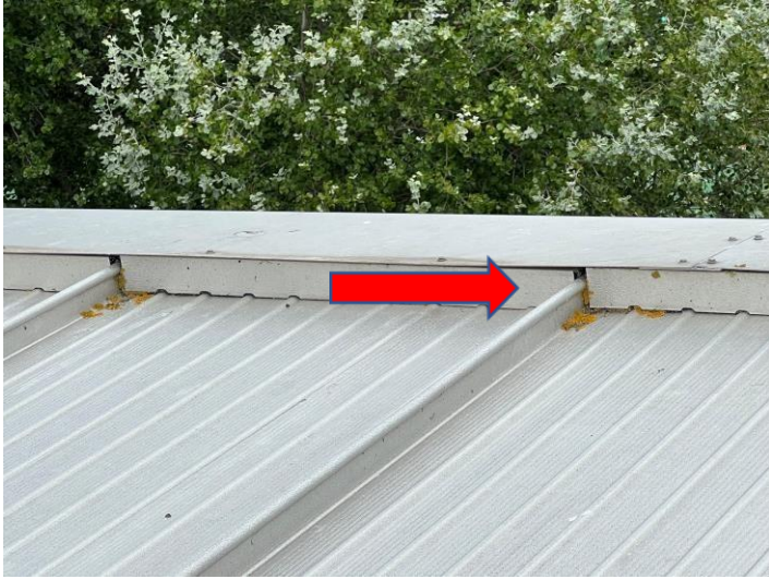
Fig 21 Gaps to infill panels
