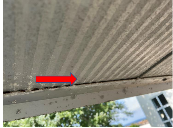
Fig 6 Delamination
