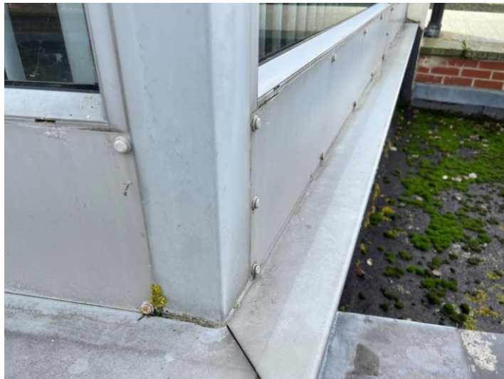
Figure 4: Connection dressing – Bridge side West
