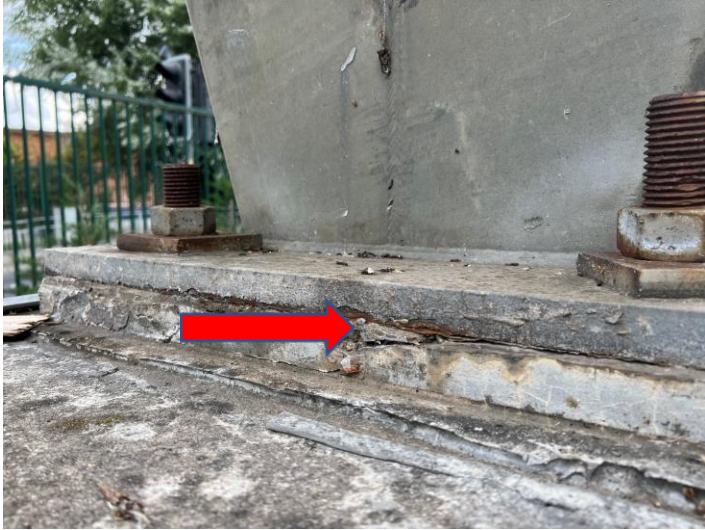
Figure 11: Light corrosion to baseplate
