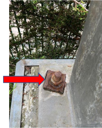
Figure 44: Moderate corrosion
