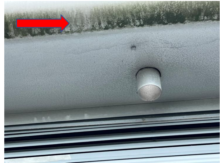
Fig 12 Moss to soffit roll
