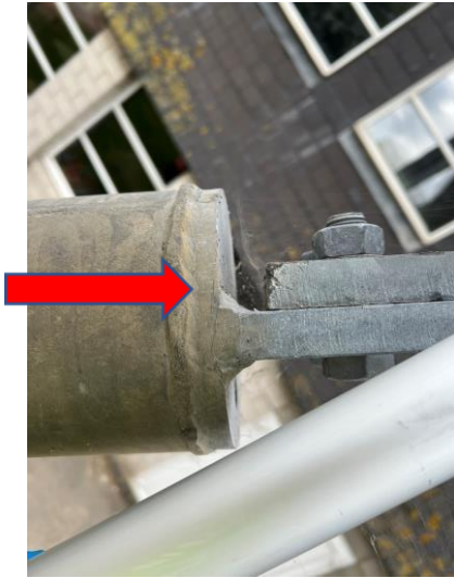
Fig 13: Light corrosion
