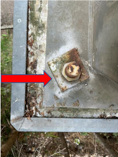
Figure 39: Moderate corrosion
