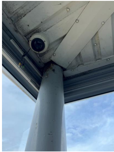
Figure 16: Upright light corrosion roof connection
