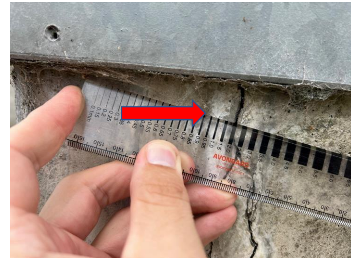
Figure 26: Degradation of grout to baseplate
