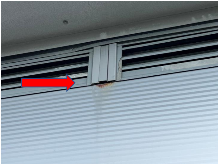
Fig 13 Light corrosion
