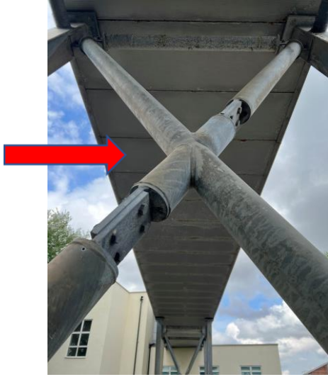
Fig 7: Pitting & light corrosion
