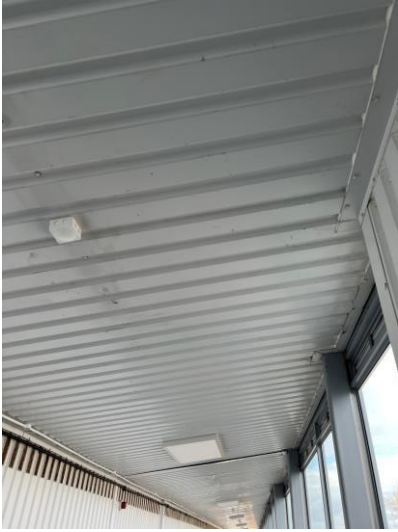
Image 5: Profiled roof deck
