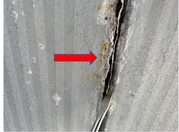
Fig 4 Heavy delamination
