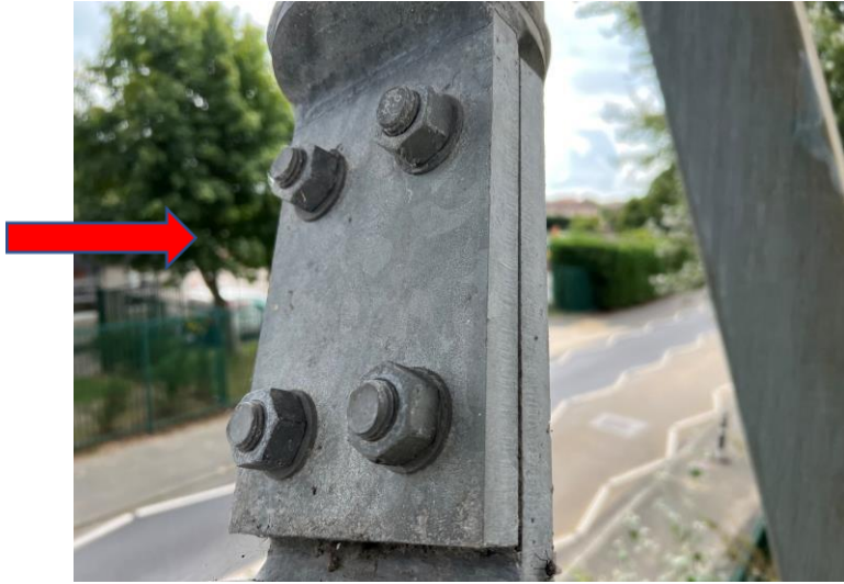
Fig 29: Connection plate
