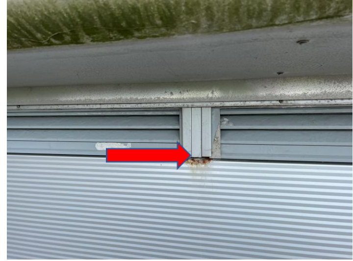
Fig 10 moderate corrosion
