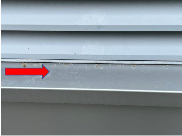
Fig 28 Light pitting to cover fillet
