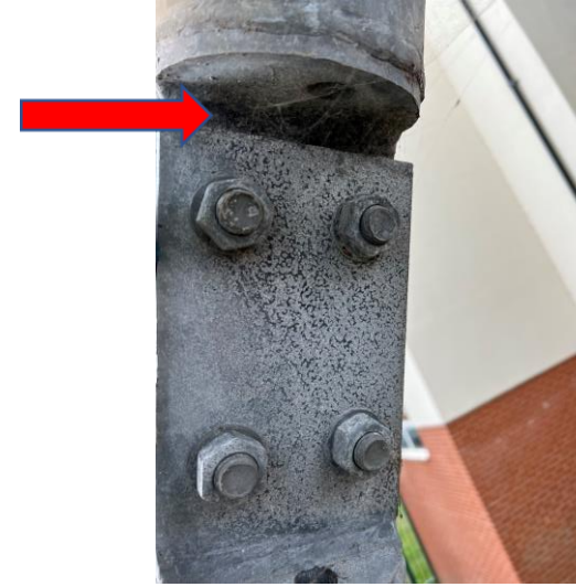
Fig 34: Pitting & corrosion
