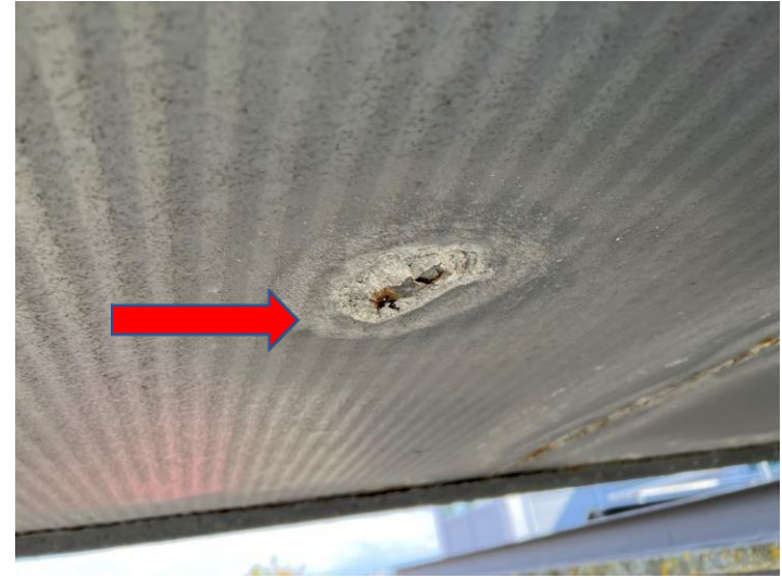
Fig 38 Heavy mid panel corrosion
