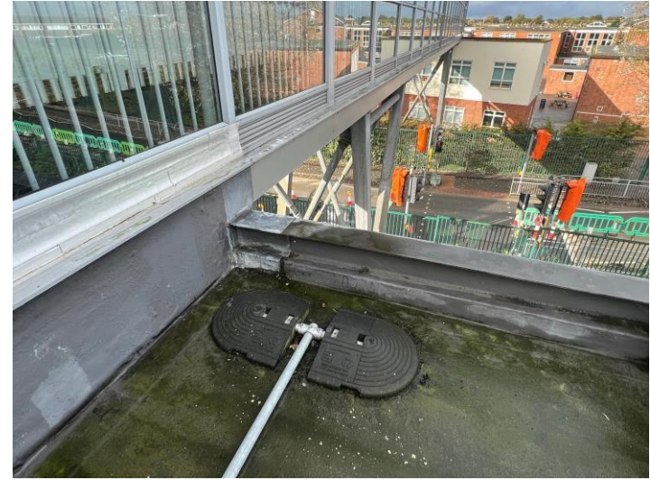
Image 16: Lack of edge protection
