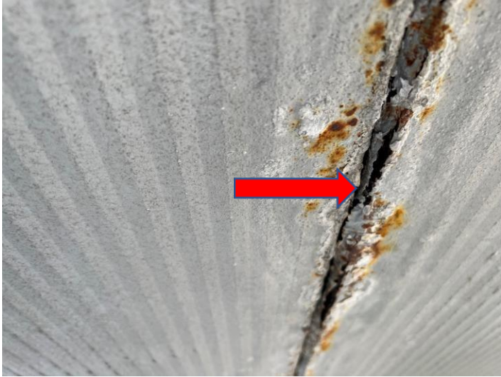
Fig 3 Heavy corrosion at joint
