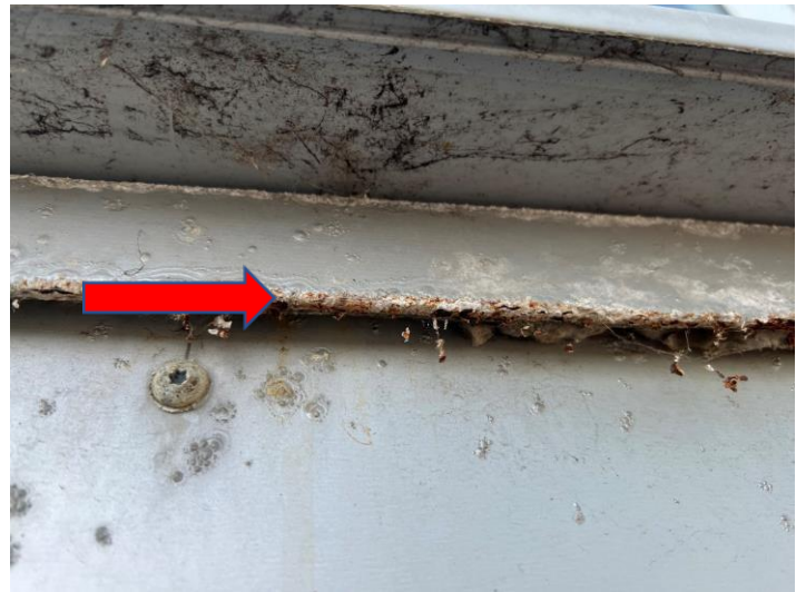
Fig 2 Light corrosion
