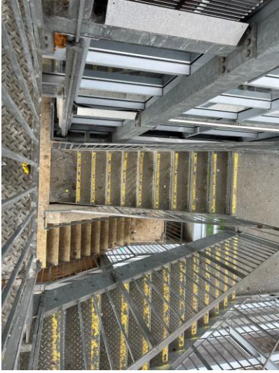
Image: Internal stair poor nosing's
