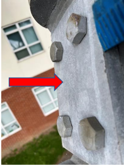
Fig 35: Connection plate
