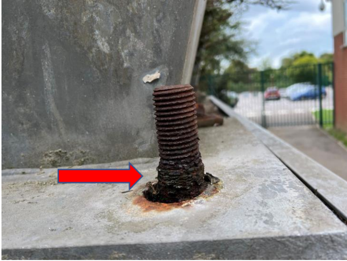
Figure 38: Moderate to significant corrosion to thread
