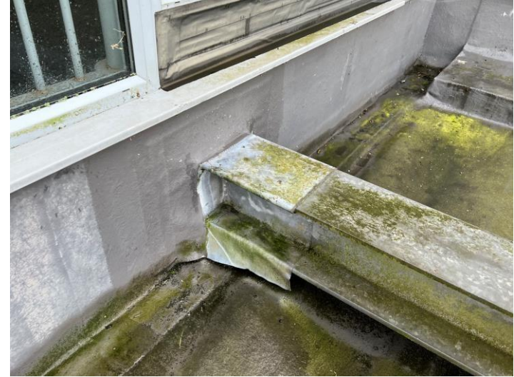
Image 22: Void & missing bird control
