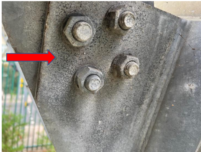
Fig 5: Light corrosion
