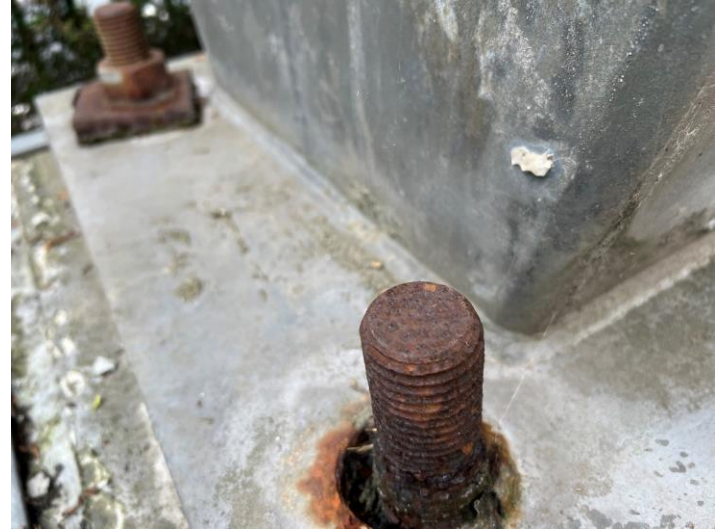
Figure 33: Light corrosion to HD Bolt & Packer
