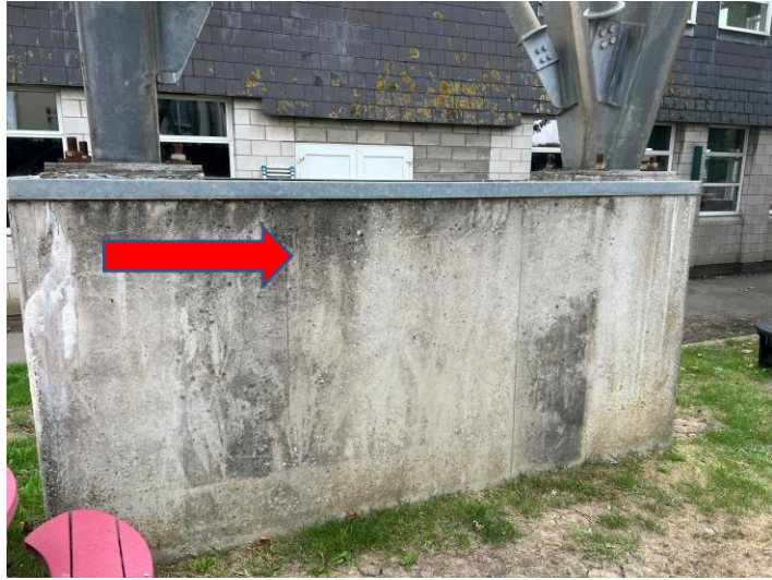
Figure 5: Staining to foundation block
