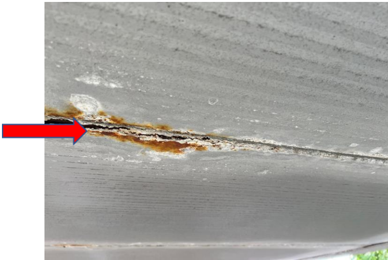
Fig 23 Heavy corrosion
