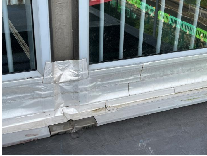
Image 7: Flash band to external cladding
