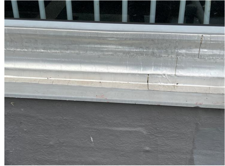
Image 8; Flash band to external cladding
