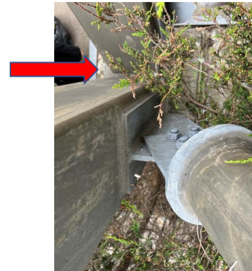
Fig 20: Light corrosion minor displacement
