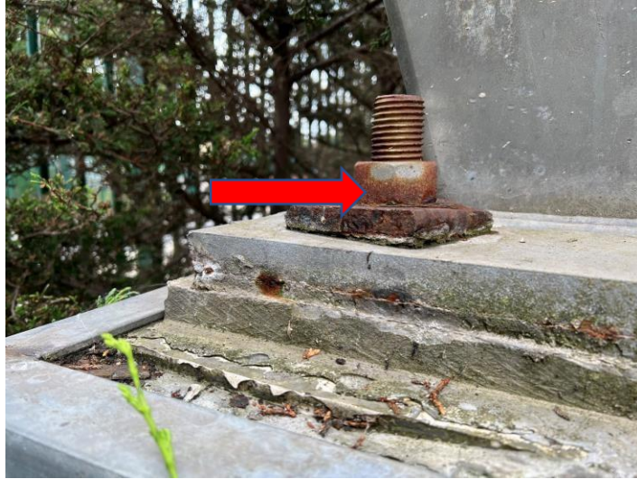
Figure 34: Missing HD Bolt West
