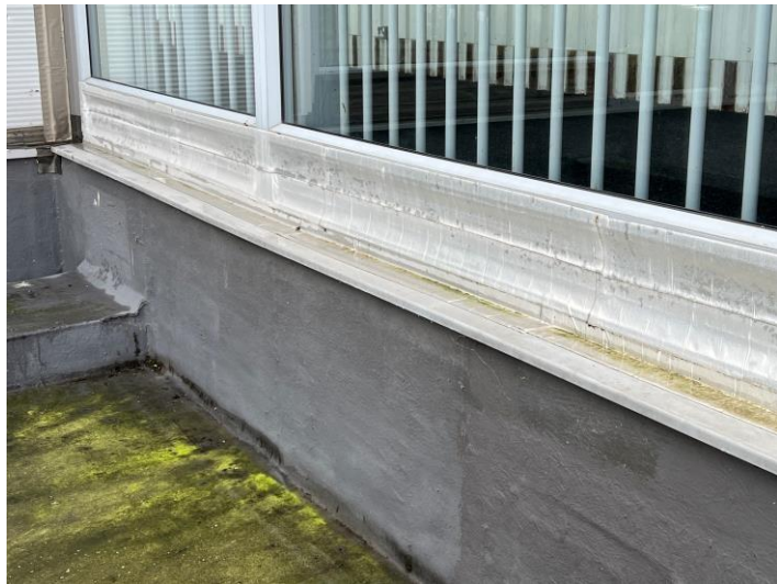
Image 7: Flash band to external cladding
