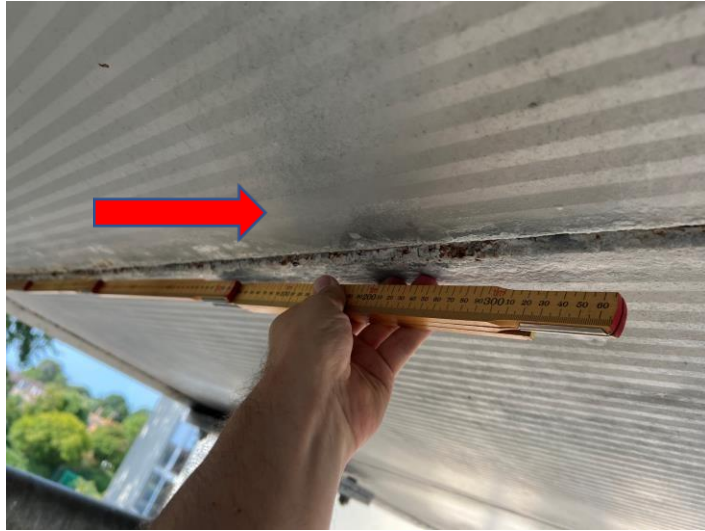
Fig 15 Moderate corrosion
