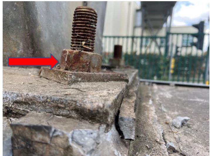
Figure 8: Degradation to grout
