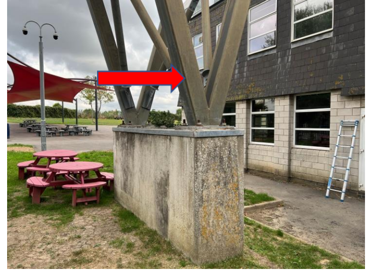
Figure 16: Light corrosion to pier
