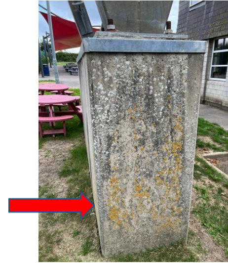
Figure 6: Moss to foundation block
