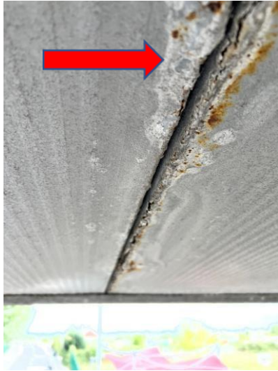
Fig 25 Delamination & heavy corrosion
