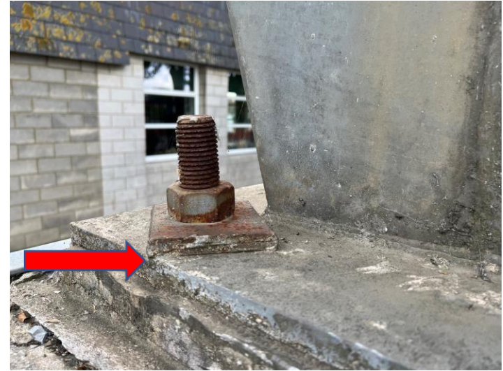
Figure 18: Moderate corrosion to HD bolt & packer
