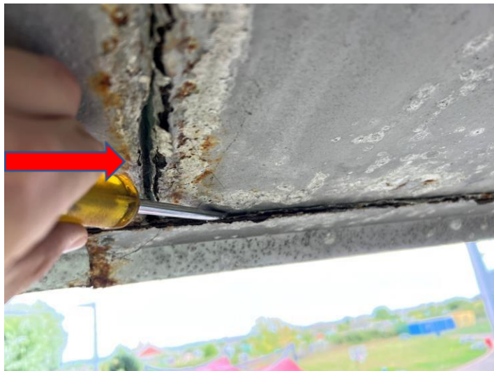
Fig 27 Delamination
