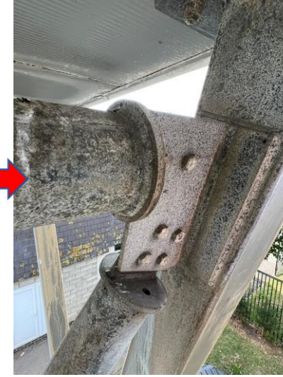
Fig 34 Moderate surface corrosion
