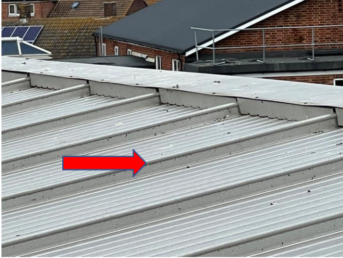
Fig 23 Rolled joints
