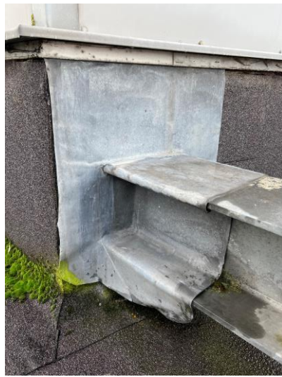
Figure 4: Connection dressing – Bridge side West
