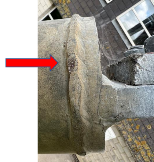
Fig 10: Light corrosion to bracing strut
