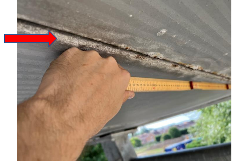
Fig 14 Moderate corrosion
