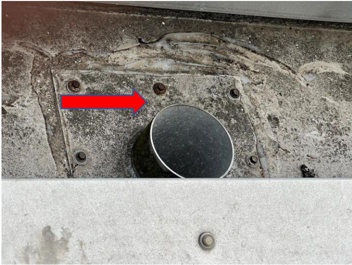
Fig 17 Proud outlet to channel
