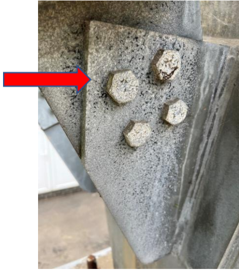
Fig 3: Pitting to connection plate
