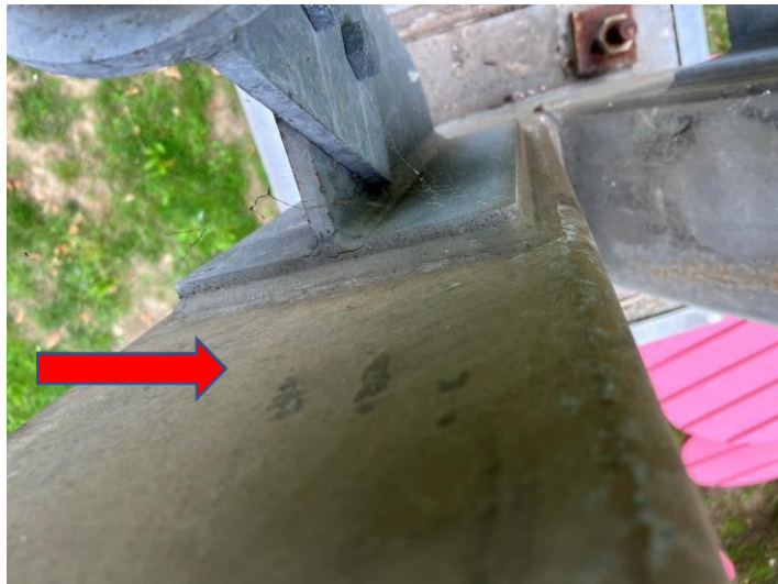
Fig 19: Light corrosion
