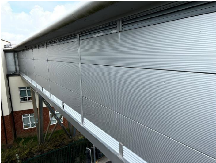
Fig 23 Rolled joints
