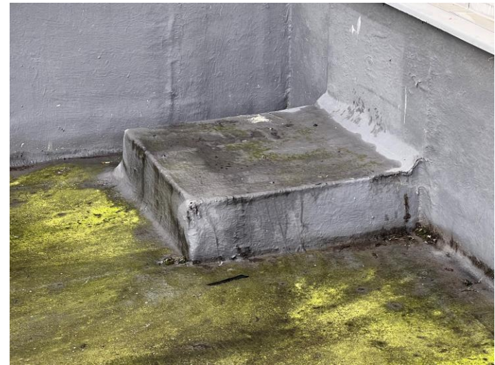
Image 8; Flash band to external cladding
