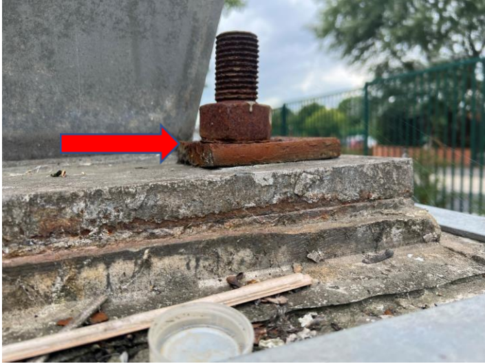
Figure 15: Moderate corrosion to HD bolt & packer
