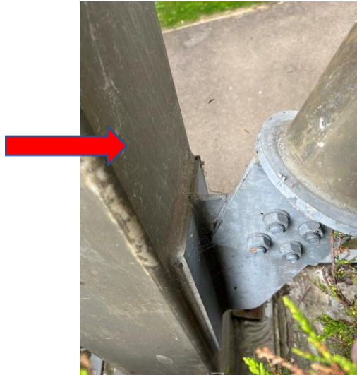
Fig 23: Light corrosion
