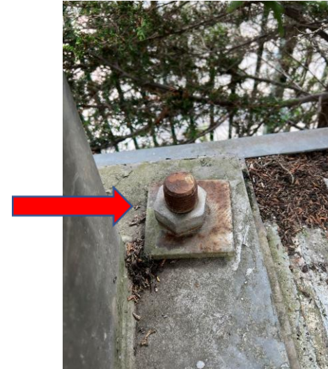
Figure 40: Moderate corrosion
