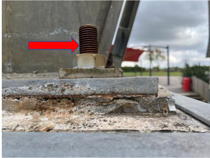
Figure 7: Corrosion to HD bolt & thread
