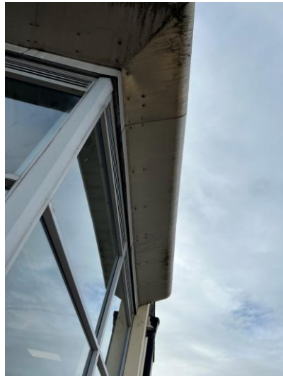
Figure 8: Staining to soffit West
