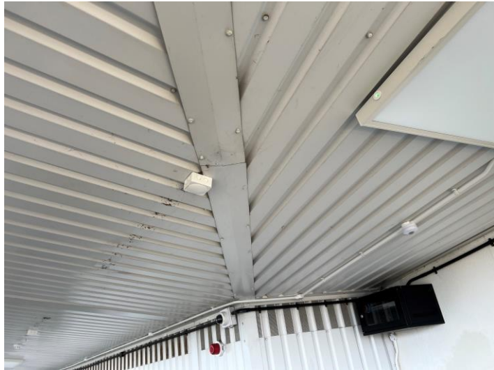
Figure 16: Upright light corrosion roof connection
