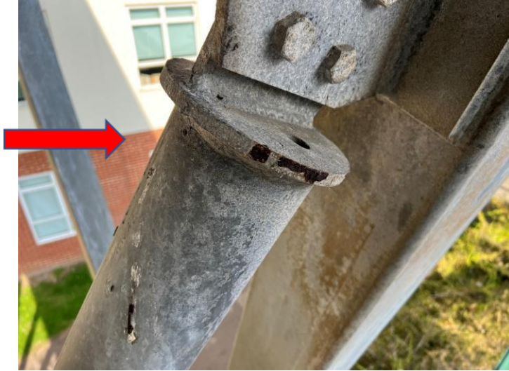
Fig 9 Moderate corrosion
