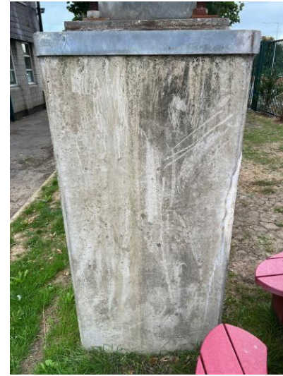
Figure 2: Foundation block East seepage
