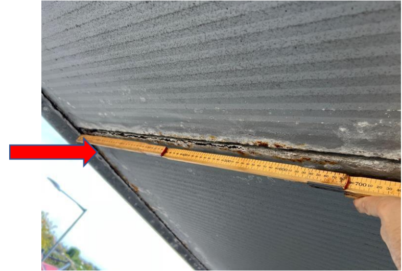
Fig 2 Heavy corrosion
