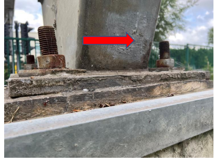
Figure 12: Corrosion to pier
