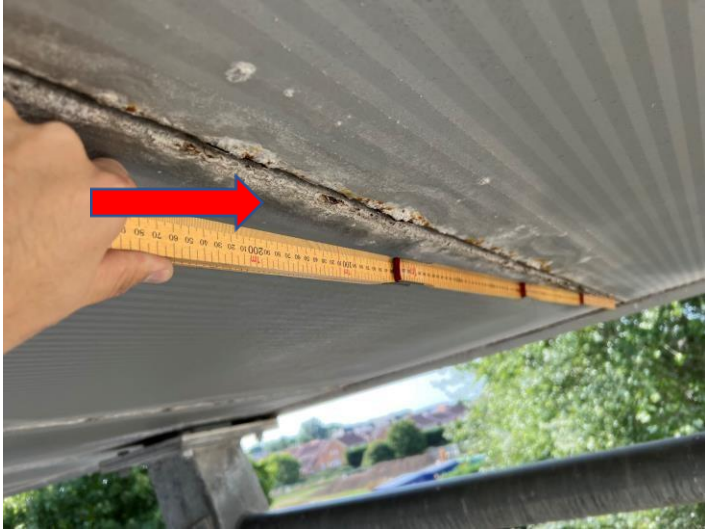
Fig 13 Moderate corrosion
