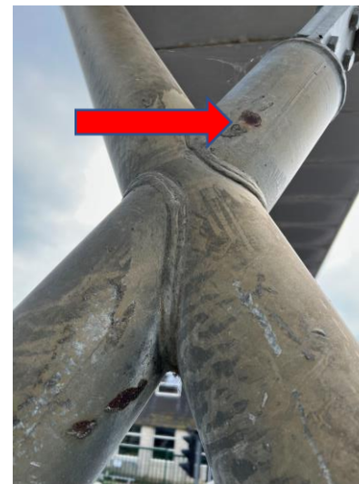
Fig 28: Strut junction light damage
