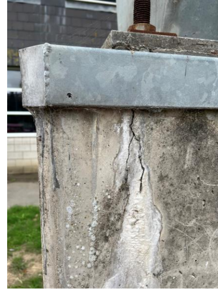
Figure 4: HD Bolt damage
