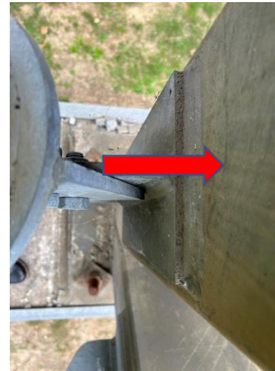
Fig 18: Light corrosion
