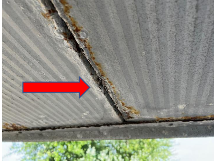
Fig 1 Moderate corrosion
