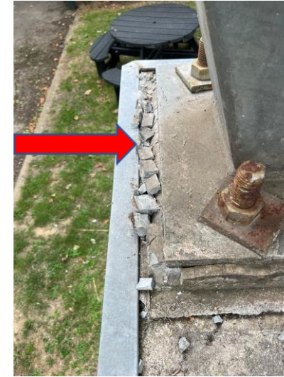
Figure 26: Degradation of grout to baseplate
