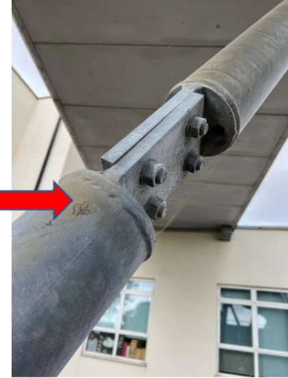
Fig 36: Light corrosion
