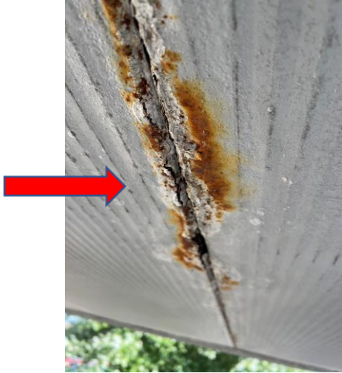
Fig 7 Moderate corrosion
