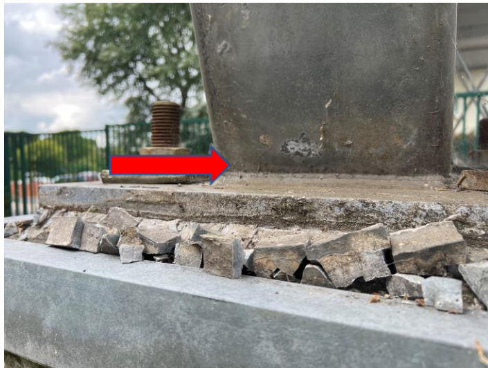
Figure 7: Corrosion to HD bolt & thread
