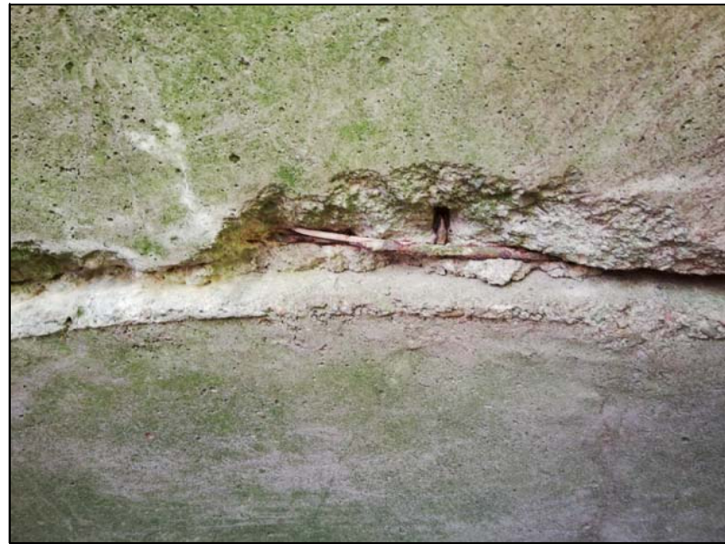
Photograph 1 - Spalled concrete with exposed reinforcement mesh
