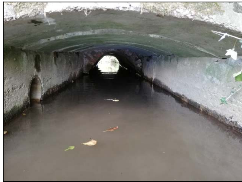
Photograph 2 - Drainage outlet within upstream north abutment
