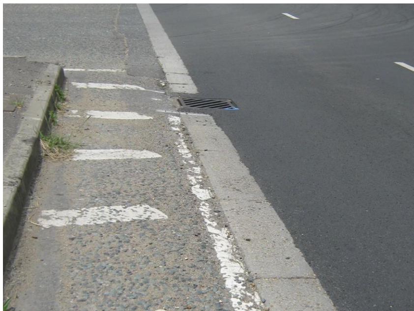
Block Type: Continuous Concrete (channel at edge of road)
