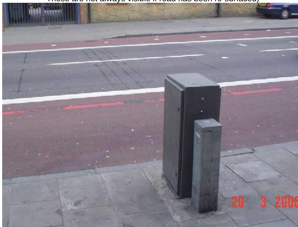
Type: Traffic Counter (Notice sealant lines in the road. These are not always visible if road has been re-surfaced)
