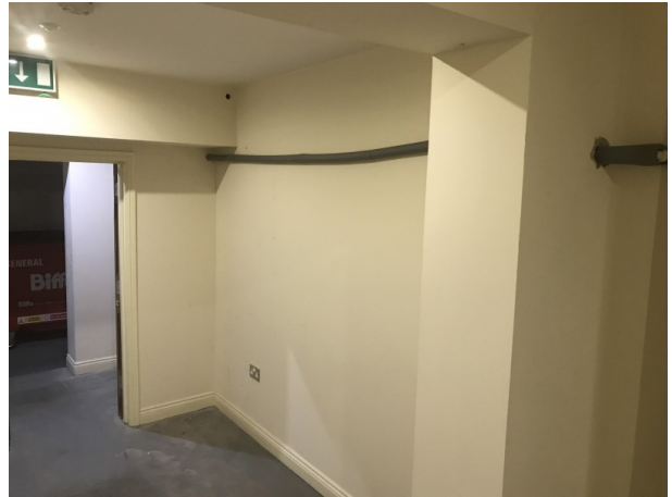
Photo - 45 Water supply to shop runs in ground floor circulation space serving flats
