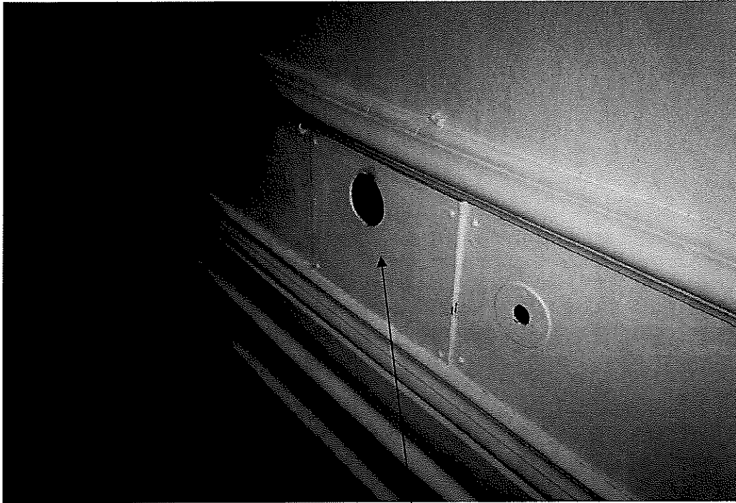
Photograph 3: Asbestos cement low level panel over ducting, level 3 De-Pass (5107/02)
