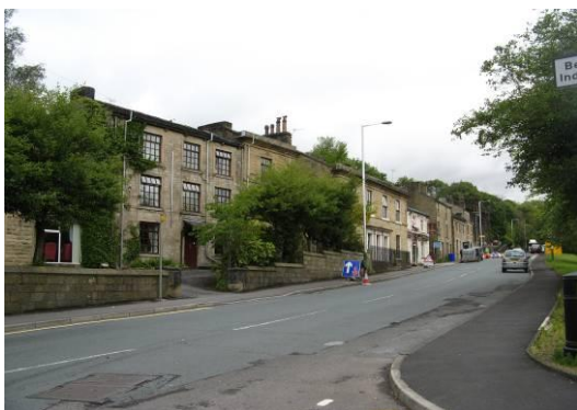
View along Todmorden Road
