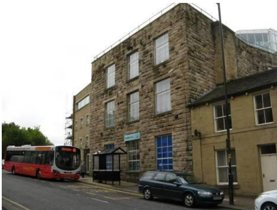
Irwell Mill, from Rochdale Road
