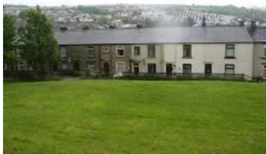
View down to Earnshaw Road
