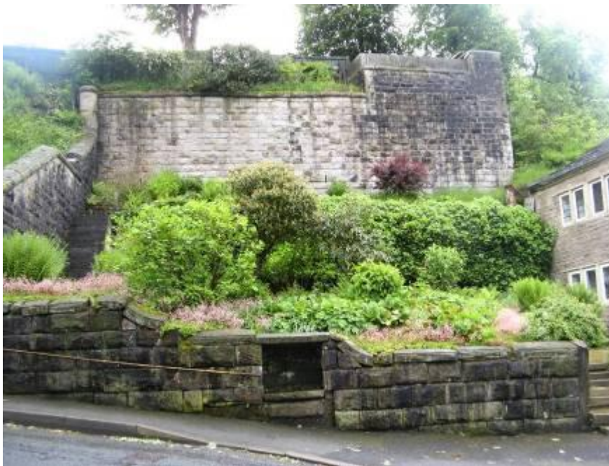
Boundary wall in Bankside Lane
