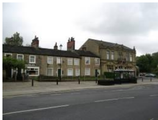
St James Street eastside
