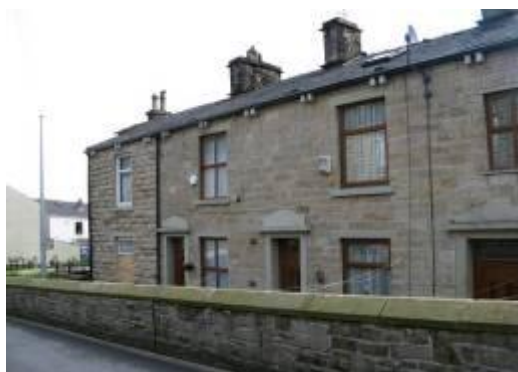
Nos. 13 and 15 Dale Street
