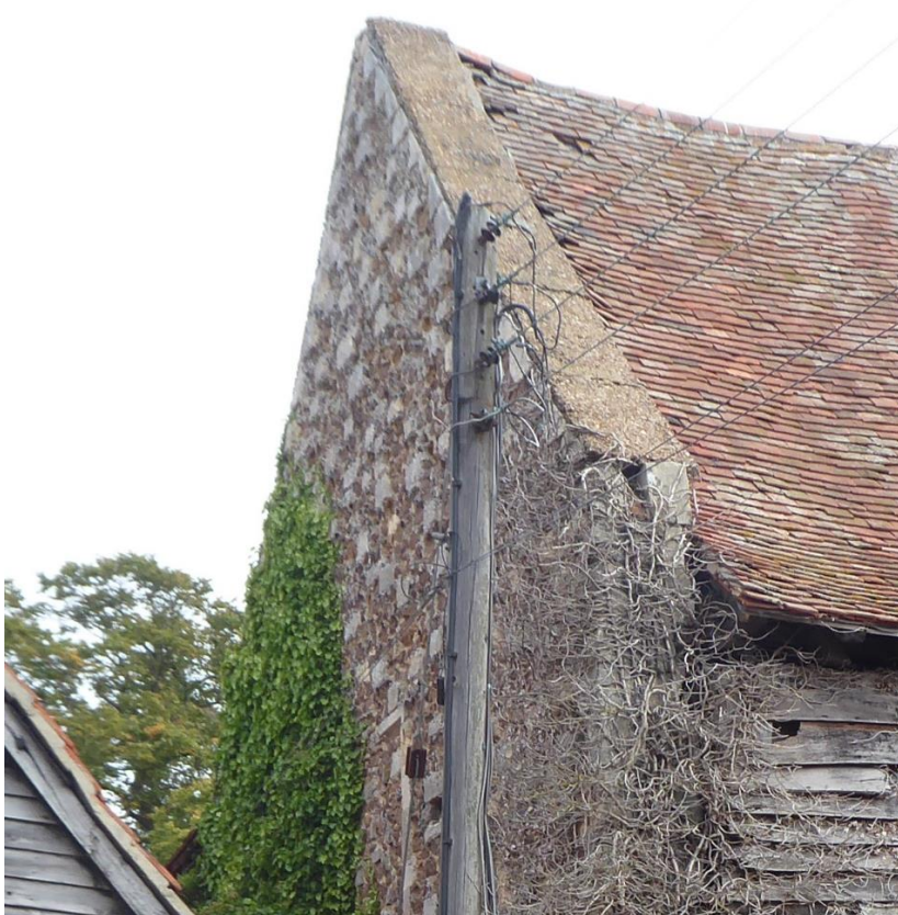
Tithe barn west wall – note rough concrete coping and live and dead vegetation
