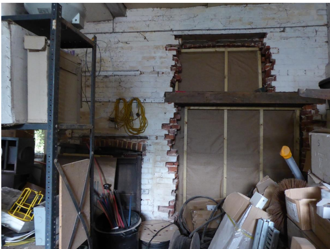
Tack room west wall – window just visible at left, old fireplace, and blocked opening
