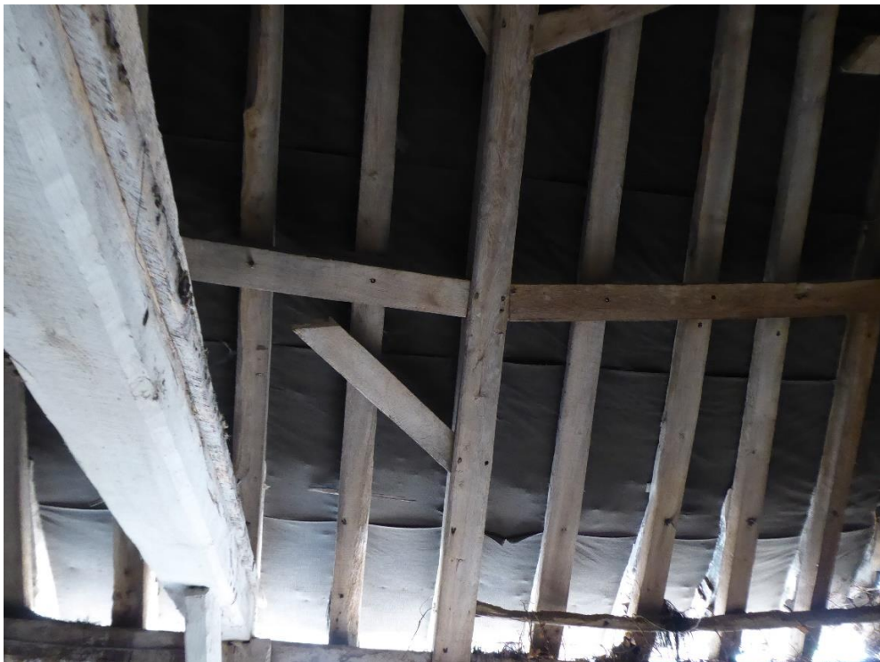
Tithe barn roof – loose brace and purlin out of line
