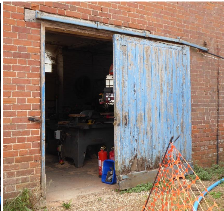
Ground floor sliding door
