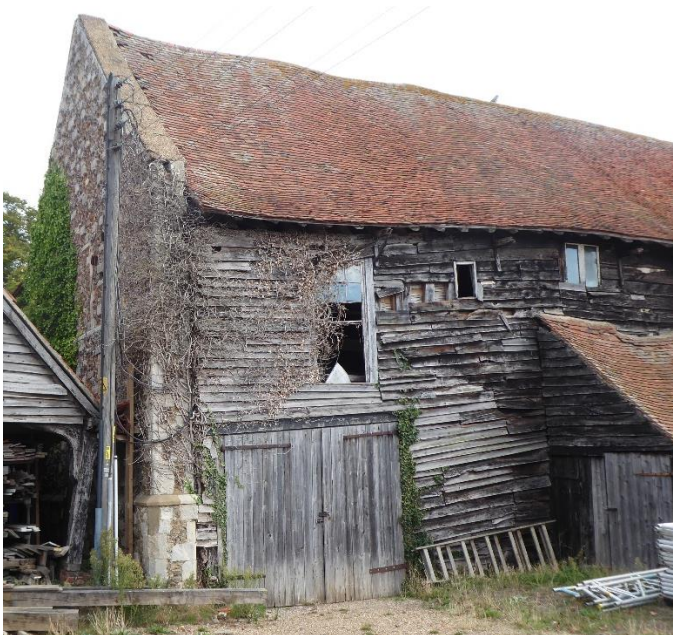
Sunk roof and wall at west end
