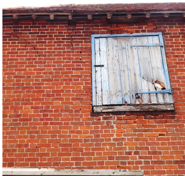
First floor door opening. Cracks are black lines on brickwork to left of doorway, but note repaired crack below the door
