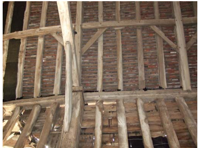
Straight-braced roof timbe
