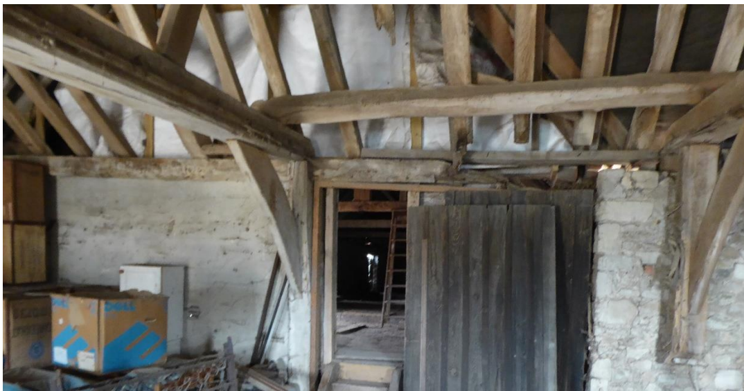
Tithe barn – damaged west end roof timbers
