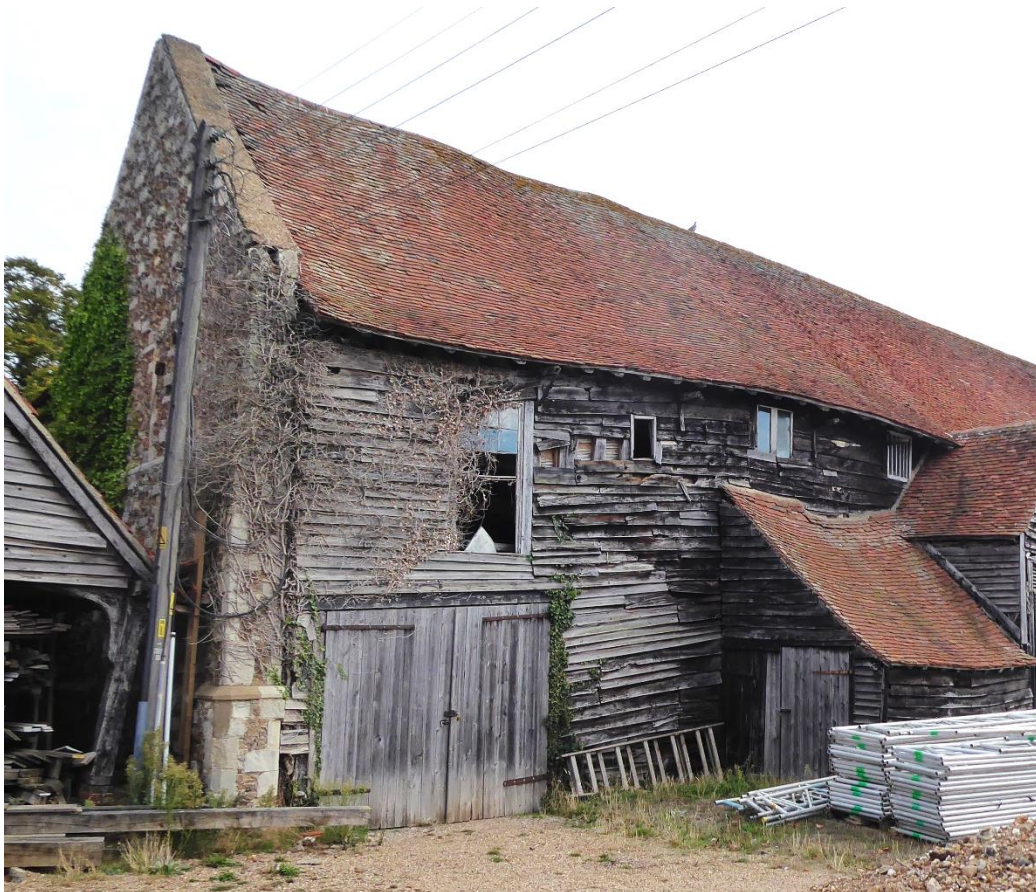
Tithe barn south wall – failed west end; note condition of window and boarding
