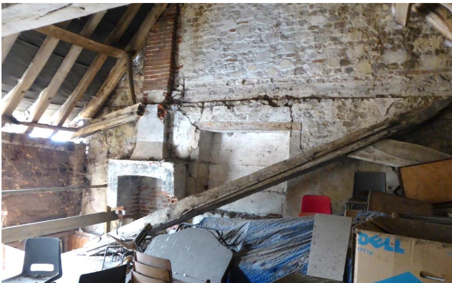
Failed tie beam at west end of roof structure
