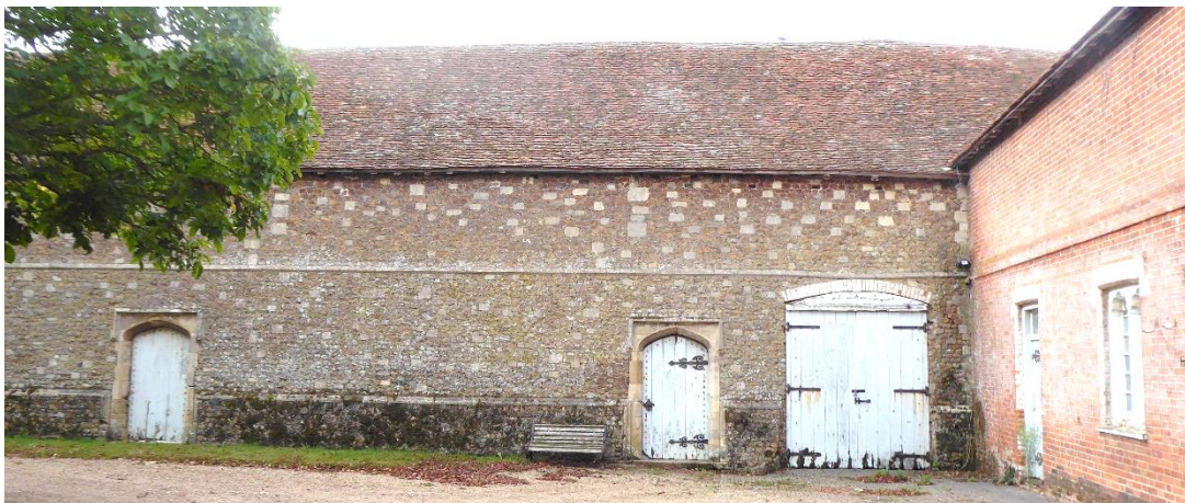
Tithe barn north wall, showing moss on plinth and decay to west cart doorway
