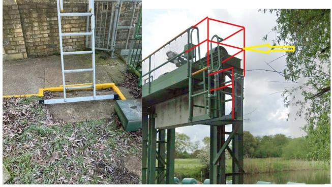
Note: The yellow arrow pointing to the rail parallel with the structure must not interfere with access when teams climb the ladder with back packs.
