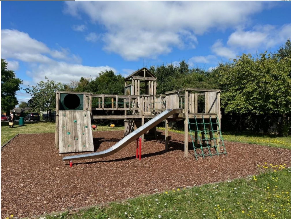
Photo Above: Unit to be removed, along with all the bark, membrane and edging. Any area not being surfaced can be topsoiled and seeded. Note the bark pit is raised in comparison to the surrounding levels.
