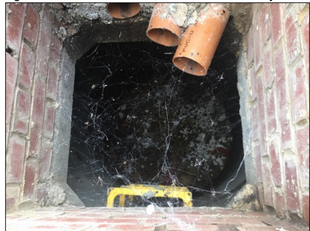
Figure 14 Main soakaway just to the north of the pavilion takes surface water from the pavilion. Depth is 3.2 m and comprises 1.2 m diameter concrete rings with a 10 course brick access.
