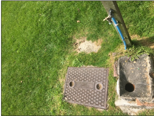
Figure 11 Potable water supply and drain into soakaway (located in NE corner of playing field).
