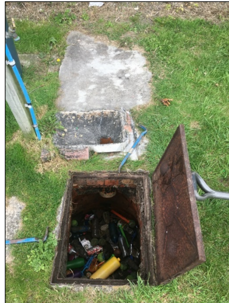
Figure 12 Connection of surface drain to soakaway.
