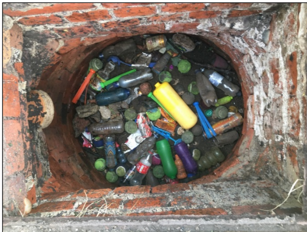
Figure 13 Soakaway is full of plastic bottle waste.
