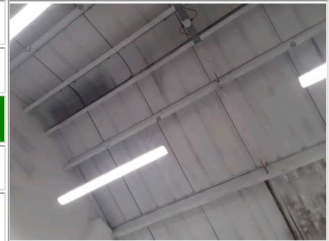
Photo No. 31 - Corrugated roof sheets (external layer - curved profile) visible to edges of skylights (as sample DE002949)
