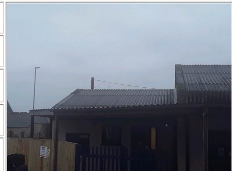
Photo No. 37 - Corrugated roof sheets (curved profile) to roof of extension to east side of building and associated edge capping panels to gable end
