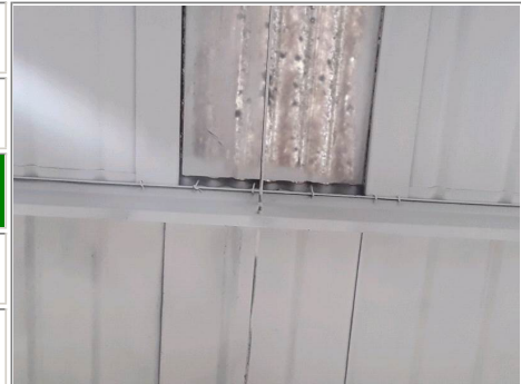
Photo No. 14 - Corrugated roof sheets (external layer - curved profile) visible to edges of skylights (as sample DE002942)
