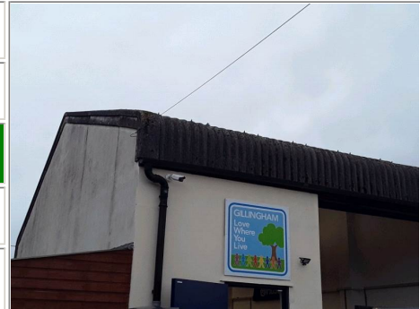
Photo No. 18 - Corrugated roof sheets (curved profile) to main roof and associated edge capping panels to gable ends (as sample DE002942)
