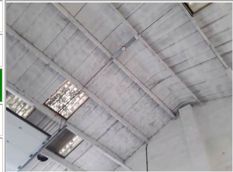
Photo No. 14 - Corrugated roof sheets (external layer - curved profile) visible to edges of skylights (as sample DE002942)
