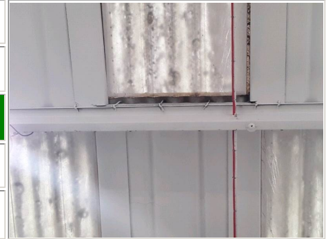
Photo No. 28 - Corrugated roof sheets (external layer - curved profile) visible to edges of skylights
