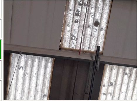
Photo No. 8 - Corrugated roof sheets (external layer - curved profile) visible to edges of skylights (as sample DE002942)
