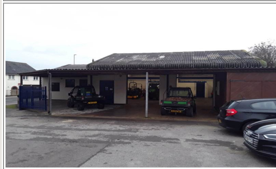
Photo No. 37 - Corrugated roof sheets (curved profile) to roof of extension to east side of building and associated edge capping panels to gable end
