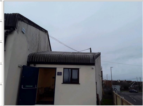
Photo No. 23 - Corrugated roof sheets (curved profile) to roof of extension to east side of building and associated edge capping panels to gable end
