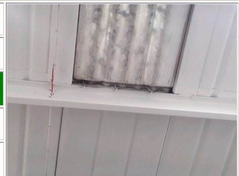
Photo No. 31 - Corrugated roof sheets (external layer - curved profile) visible to edges of skylights (as sample DE002949)
