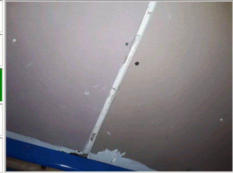
Photo No. 16 - Textured coating to original ceiling above new plasterboard ceiling panels (visible via small gap between new plasterboard ceiling panels) (as sample DE002933)
