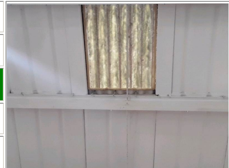
Photo No. 2 - Corrugated roof sheets (external layer - curved profile) visible to edges of skylights
